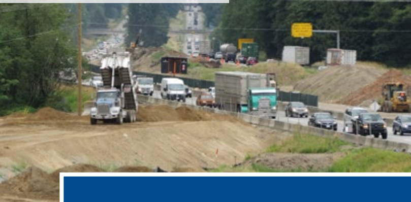
Building westbound exit ramp
