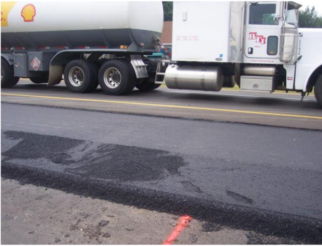
B7 - Sampling hole filled up with new asphalt mix.
