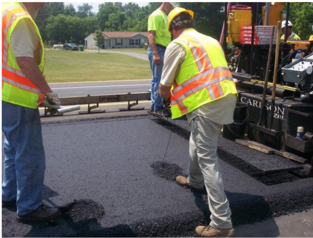
B3 - Locating sampling plate with attached wire after asphalt mix is placed.
