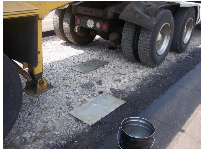
B2 - Plates prior to placement of asphalt mix by paver.
