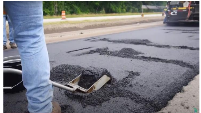
A2: Lifting shovel full of asphalt mix.
