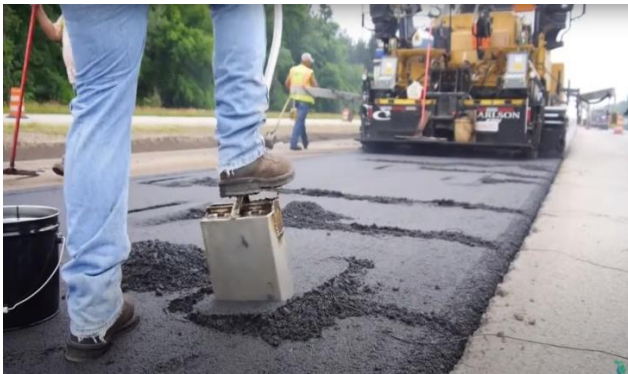
A1: Digging Shovel directly into asphalt at selected location.
