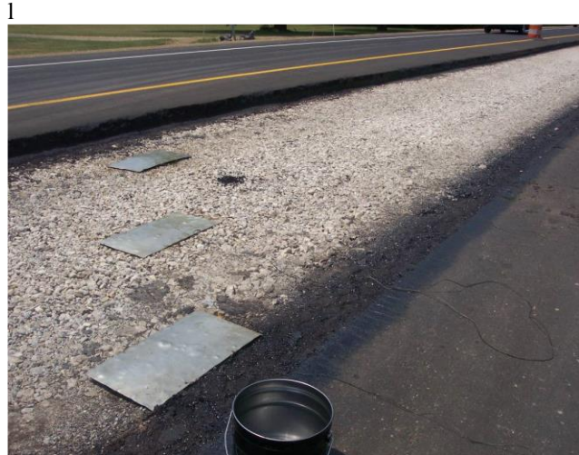
B1 – Placing sampling plates on the existing surface.
