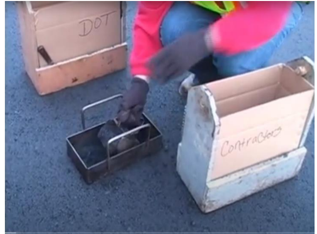
C4 - Removing asphalt mix inside the sampling template using scoop.
