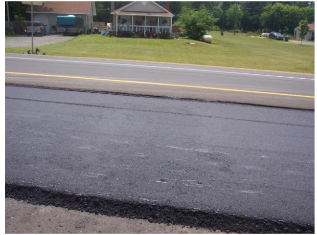
B8 - Sampling location after placement of new mix and compaction.
