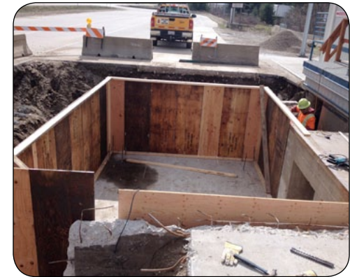
Work underway in Castlegar to install heated and enlarged scale pit.
