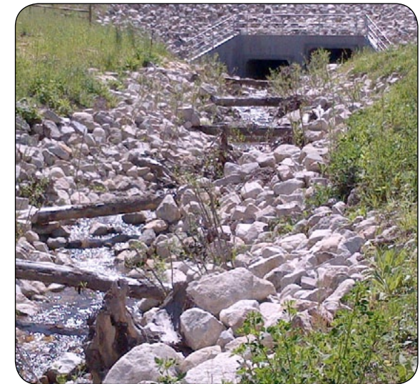
Willow stakes adjacent to the stream and logs placed in the stream provide shade, nutrient sources and improve fish habitat.
