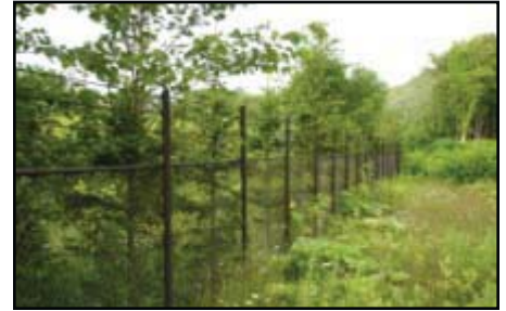
Shari Eco-Road wildlife exclusion fencing
