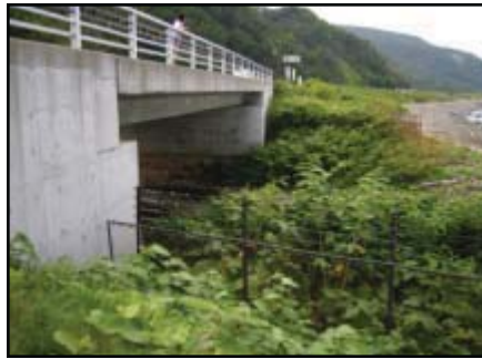
Shari Eco-Road wildlife underpass
