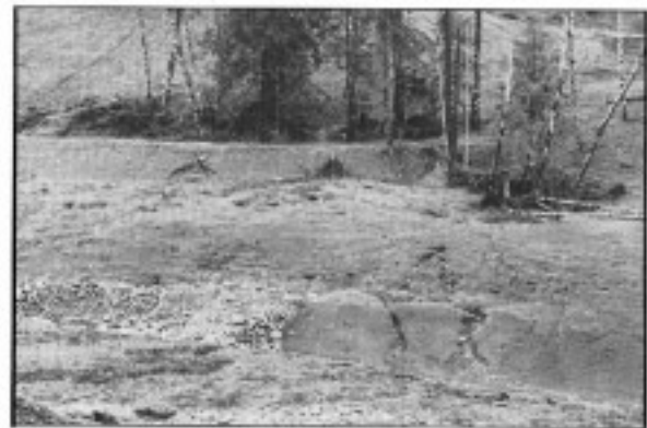
Fig. 15. A waste area with a protection dyke.
