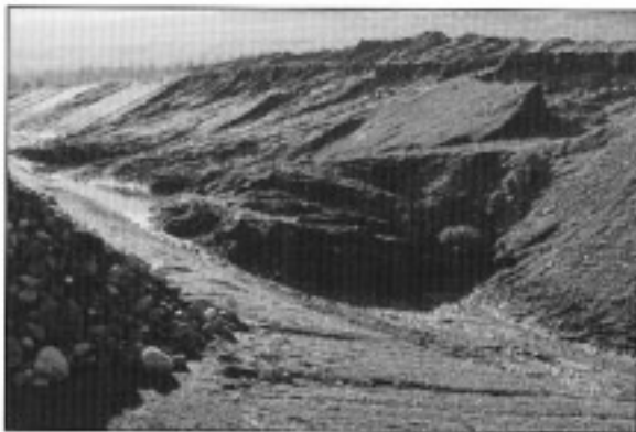
Fig. 11. Shallow slope movement into a ditch, leading to more erosion.
