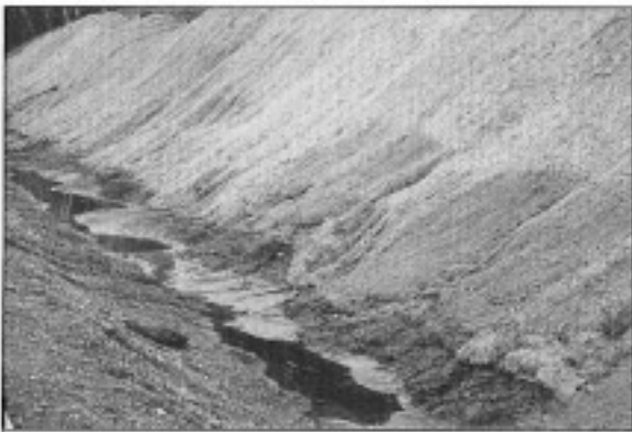
Fig. 20 Erosion under a manufactured blanket.
