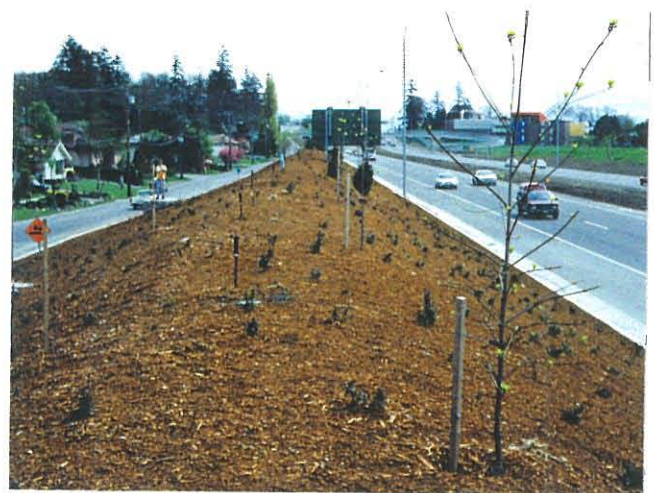
Figure 3.3; A 4 m High Berm with a 1.5 m Wide Quasi-flat Top, Between Pat Bay Highway and Douglas St. near Victoria
