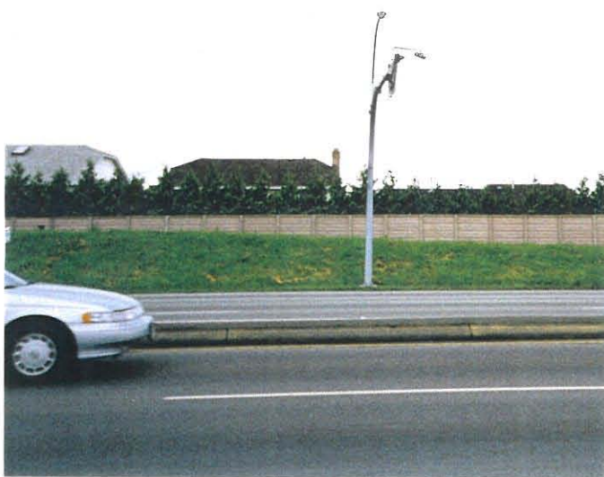
Figure 4.1; Transition from a Pure Wall to a Pure Berm via a Berm/Wall Combination - Highway 17 near Highway 10, Delta.
