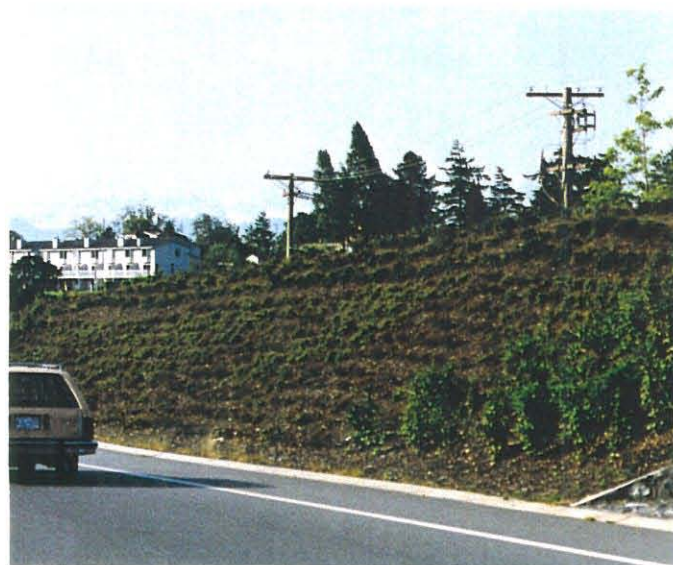
Figure 4.3; A Relatively Sound absorptive Berm Near the McKenzie Interchange, Victoria
