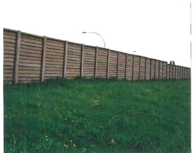
Figure 2.5; A 3 m Berm/1.5 m Wall Combination Noise Barrier along Highway 17 in Delta
