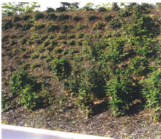
Figure 5.2; A Berm Dressed with Bark Mulch and Planted with Small Bushes and Shrubs
