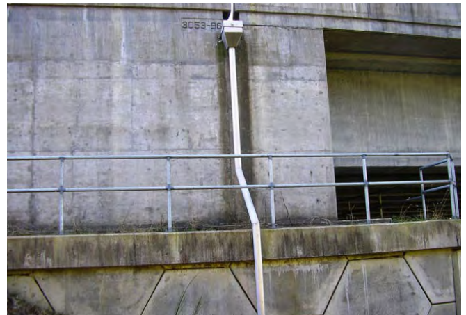
Photo 10. Collection downpipe at outside of bridge expansion joint.
