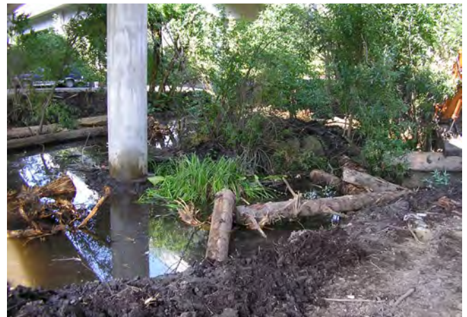
Photo 12. Constructed habitat pond underneath bridge. Additional benefits of reducing vegetation maintenance and bridge over ponds provides cover and shade for coldwater fish species.
