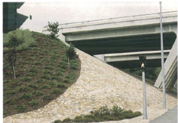
Figure H-21 Example of a more urban bridge abutment.
