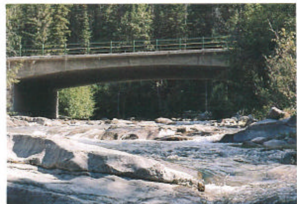
Figure H-5 Bridging streams whenever possible is preferable to installing culverts. Bridges maintain the continuity of the watercourse and help to minimize the impact of highway construction on natural systems.
