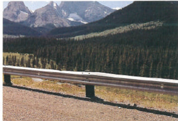
Figure H-29 Consider installation of "see-through" forms of traffic barrier where views below the highway are frequent.
