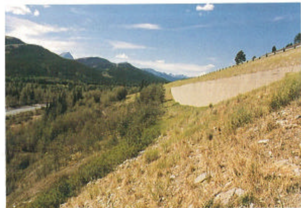
Figure H-24 Viewed from the road this retaining structure is completely hidden.
