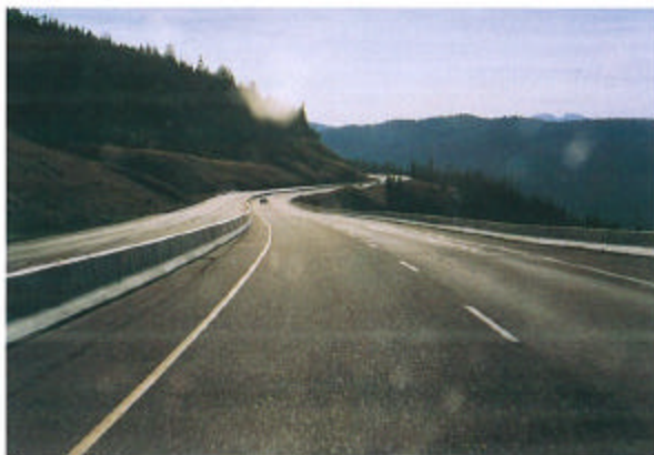
Figure H-26 The provision of a wide and varied median could have avoided the requirement for a continuous traffic barrier.
