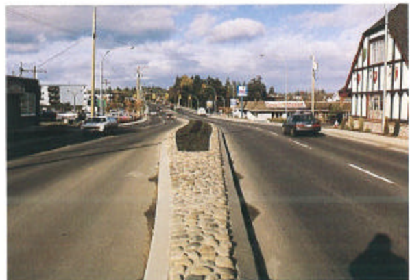
Figure H-38 Decorative paving should be installed in traffic islands and medians where space is insufficient to allow planting.
