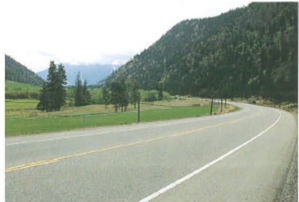
Figure B-1 Example of a rural Baseline Highway.
