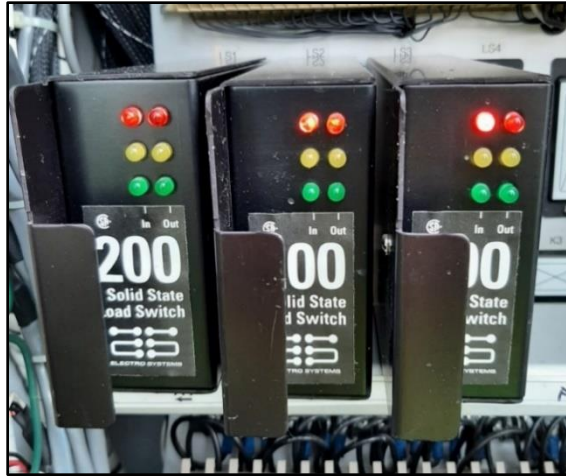
Figure 6. Cabinet Load Switches
