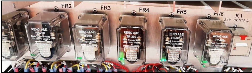
Figure 11. 'P6' Flash Transfer relays
