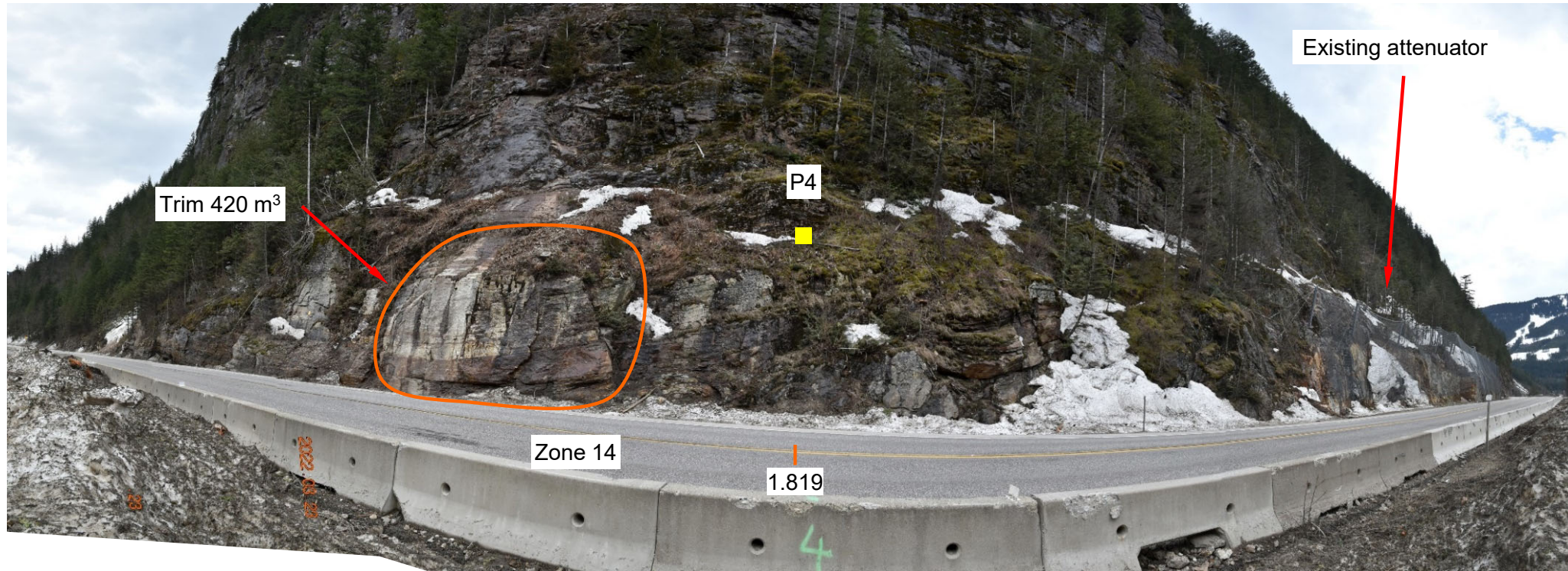
Photos #9: View of site showing location of proposed work
