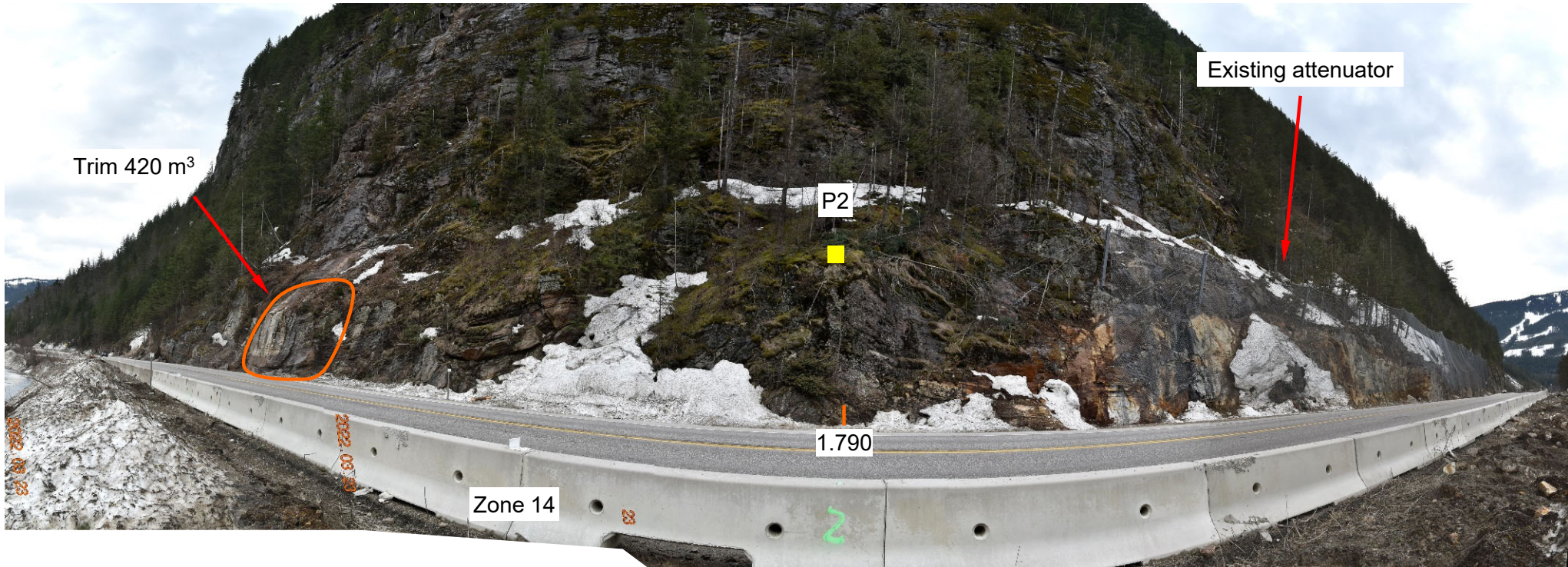
Photos #7: View of site showing location of proposed work
