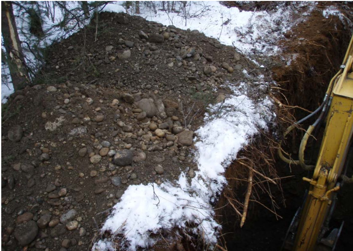
Photo # 10. Pit Run Materials – TP07-25
