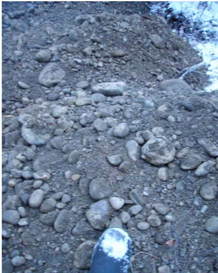
Photo # 15. Pit Run Materials – TP07-30
