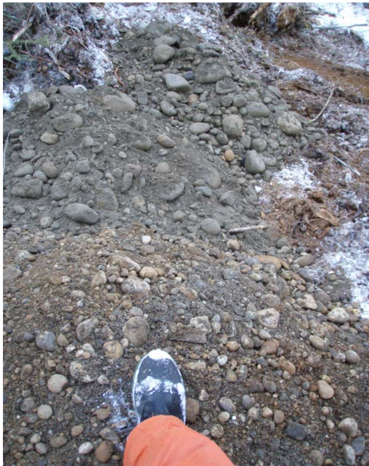
Photo # 4. Pit Run Materials – TP07-18
