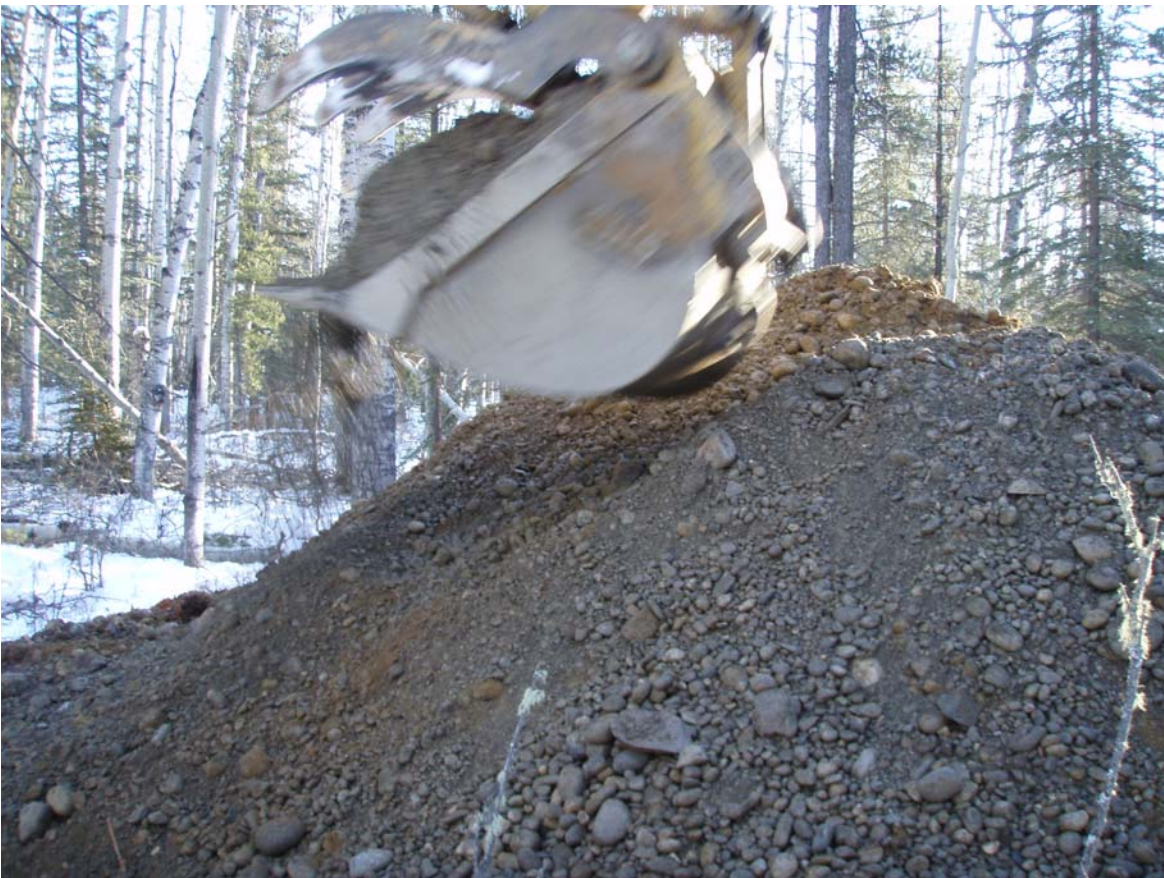
Photo # 2. Pit Run Materials – TP07-11
