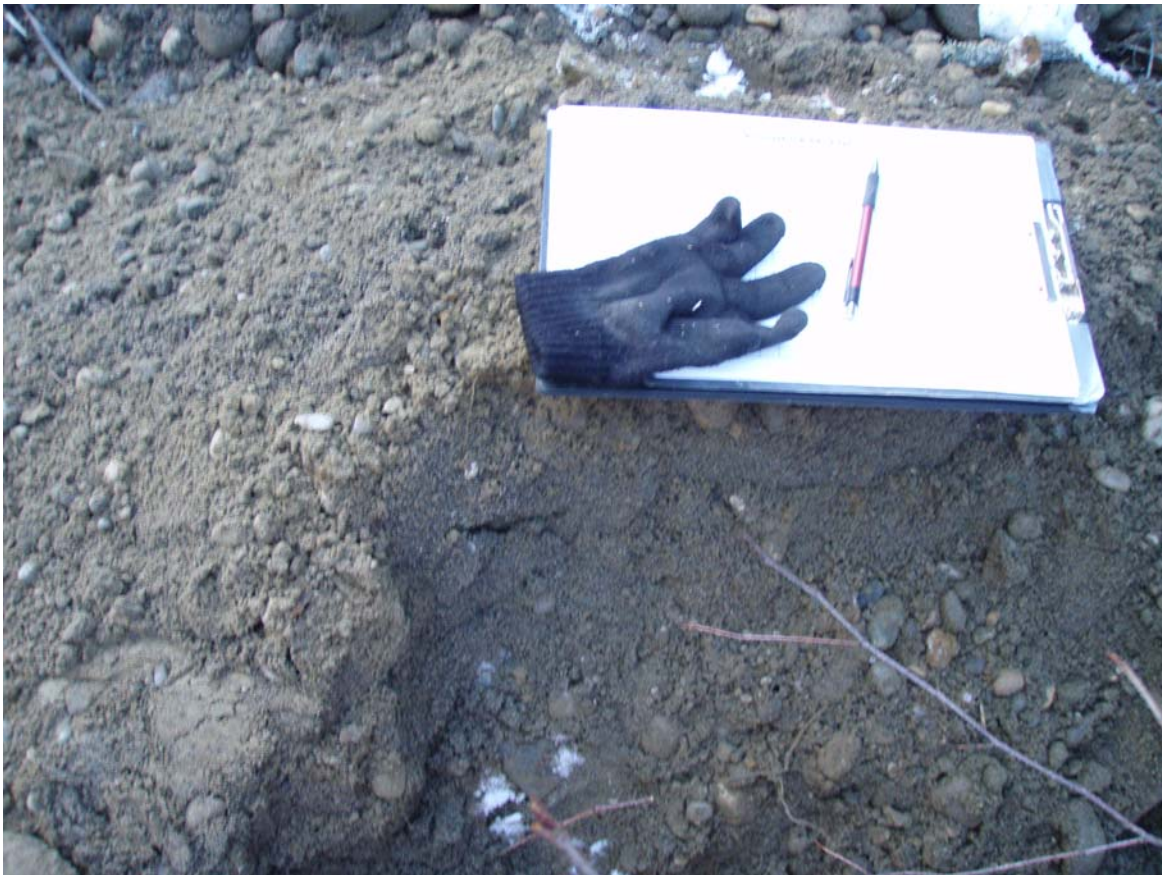
Photo # 7. Pit Run Materials – TP07-21
