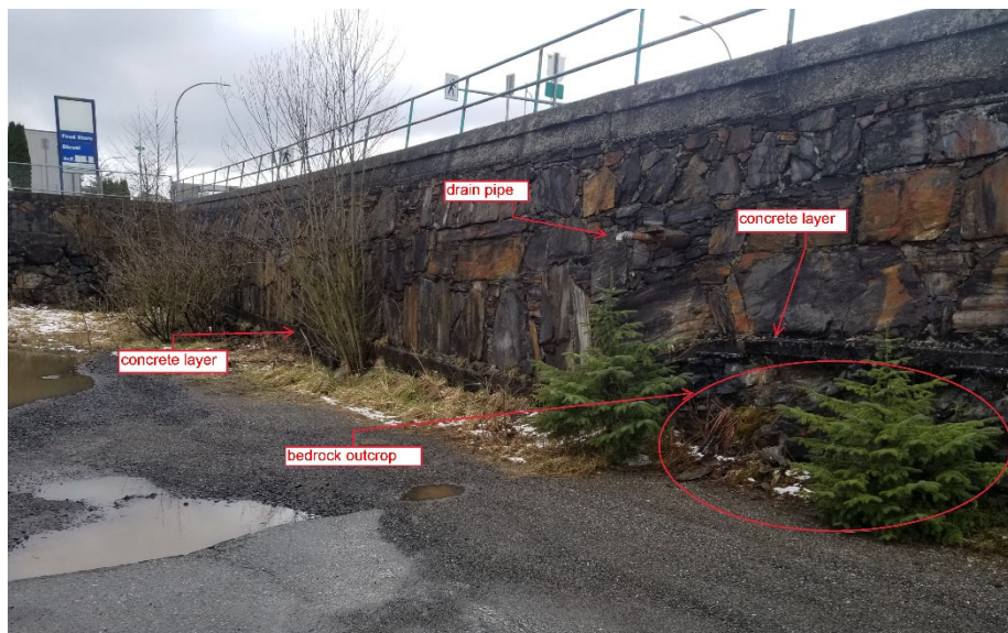
Figure 4: View of rock wall along 2 nd Ave W looking south approximately mid way along the wall.
