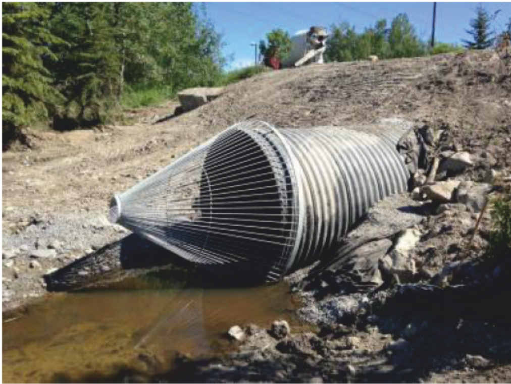
Figure 6-2: Beavercone Product Installed at Culvert Inlet to Prevent Debris Clogging (Fleming, 2022)
