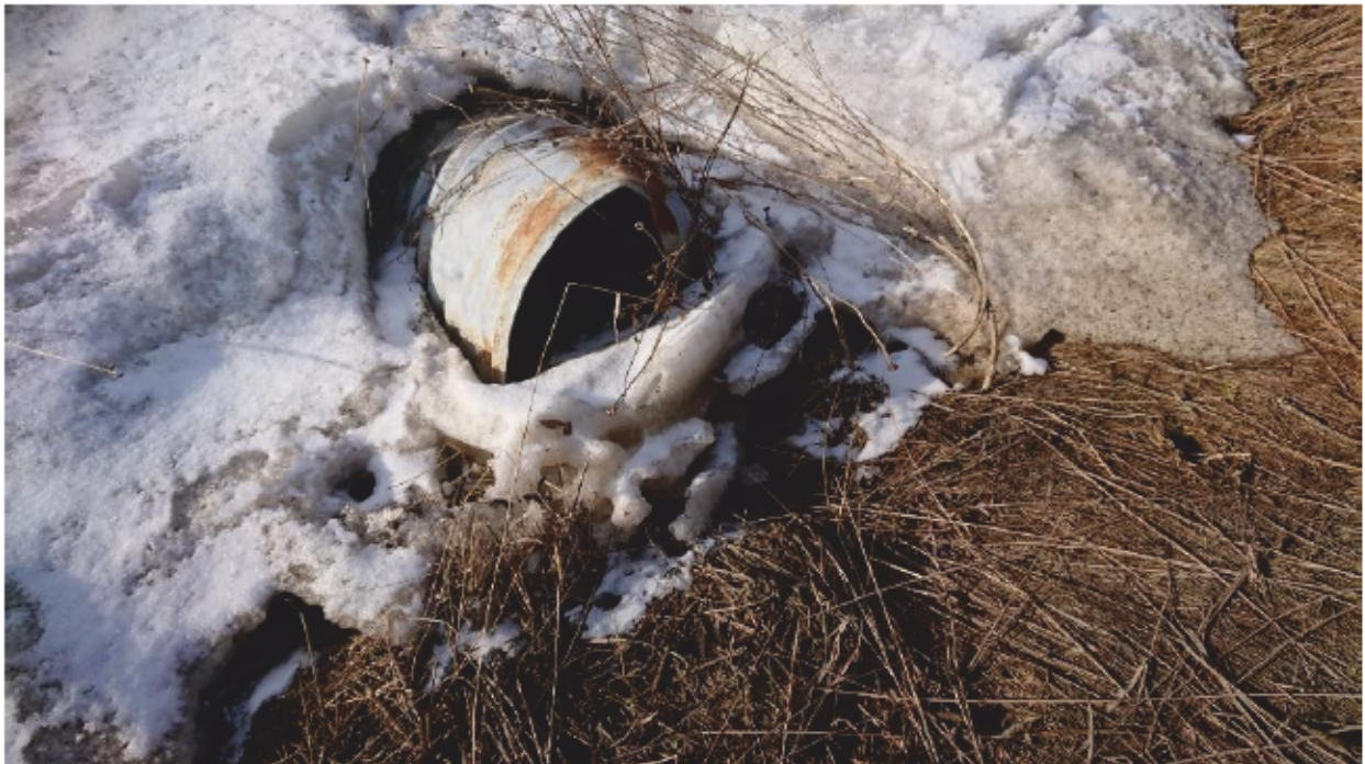
Figure 2-6: Existing 450mm Culvert Inlet at Sta. 601+42
