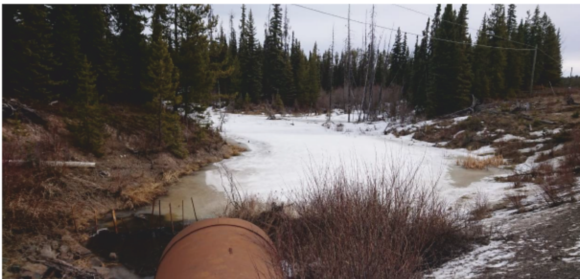
Figure 2-2: Pond upstream of the Main Culvert Crossing in March 2021 (Sta. 104+91)
