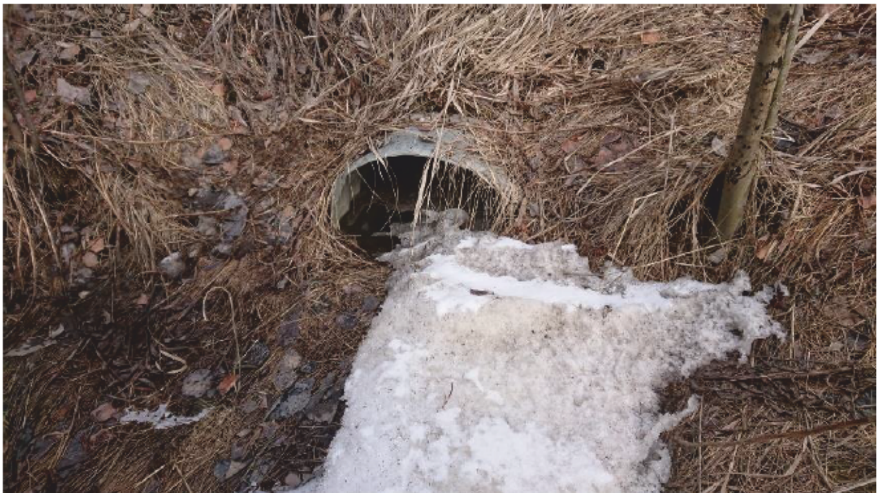
Figure 2-10: Existing 450mm Culvert Outlet at Sta. 600+95
