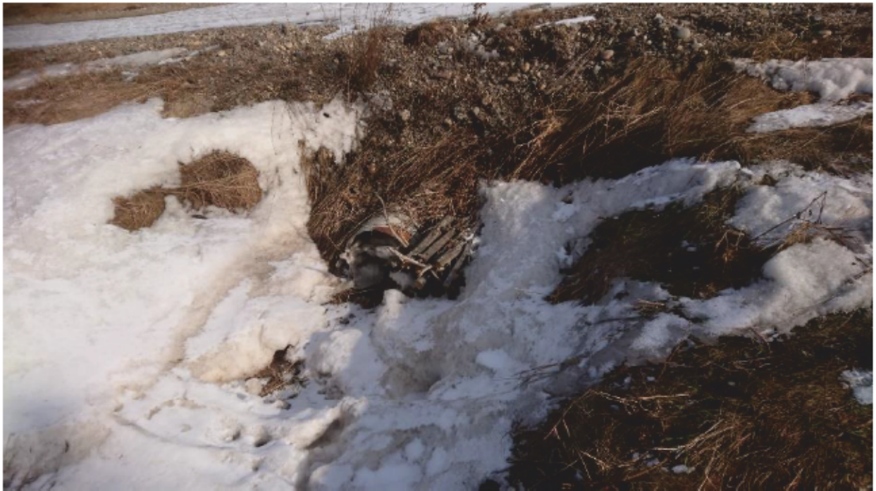
Figure 2-5: Existing 450mm Culvert Outlet at Sta. 601+42
