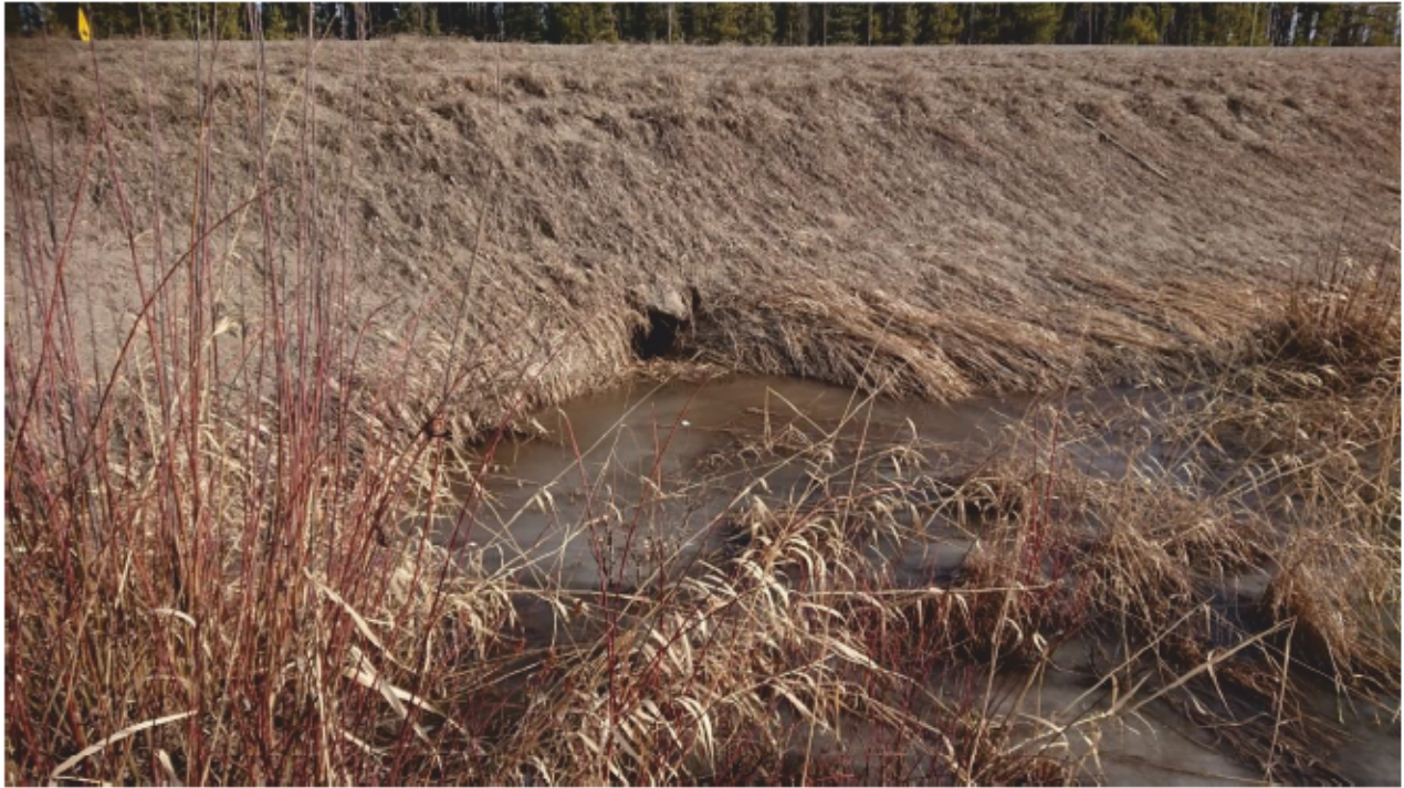
Figure 2-9: Existing 750mm CSP Culvert Inlet at Sta. 107+48
