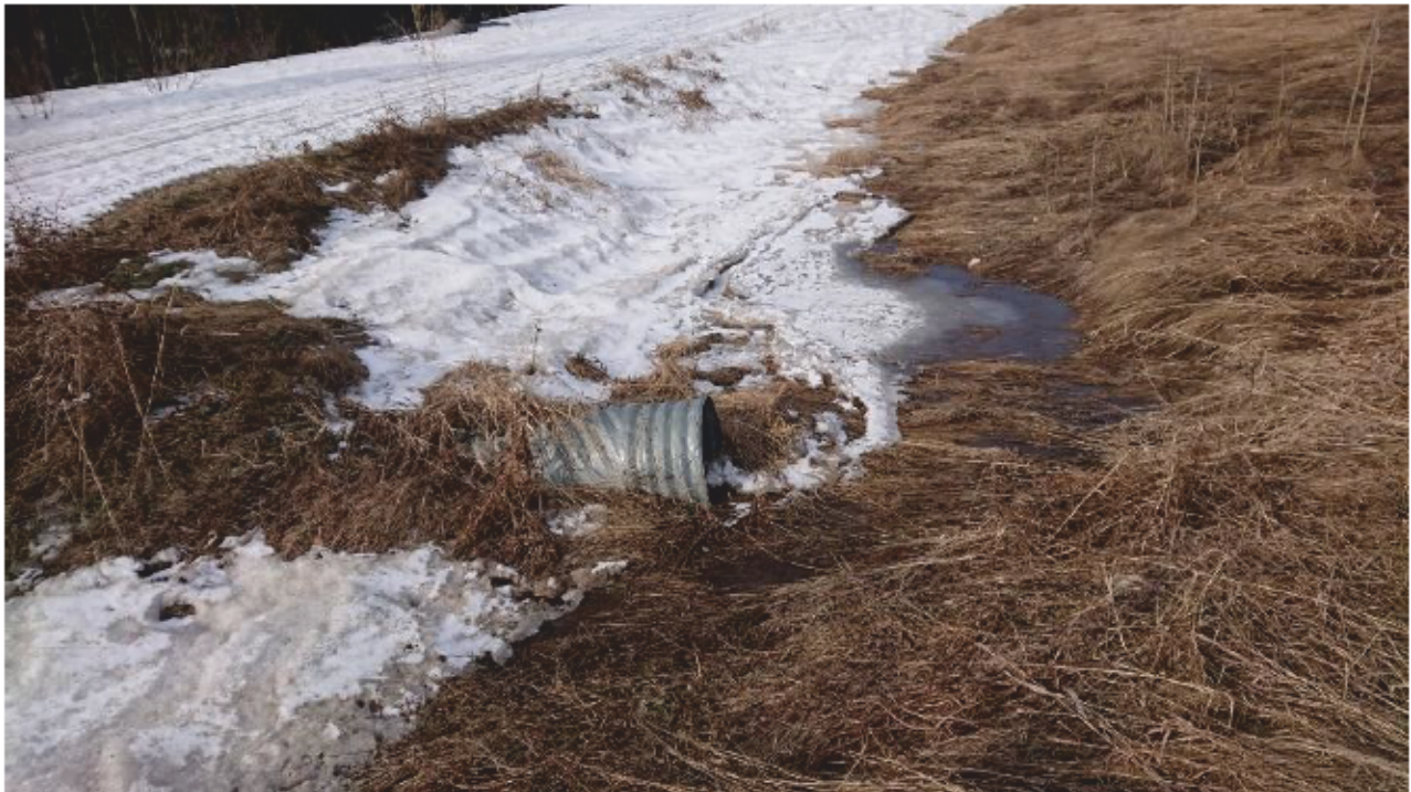
Figure 2-11: Existing 450mm Culvert Inlet at Sta. 600+95
