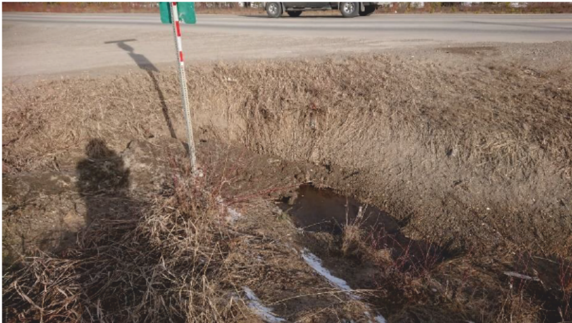
Figure 2-7: Existing 450mm Culvert Inlet at Sta. 700+10 (Shallow Bay Road)
