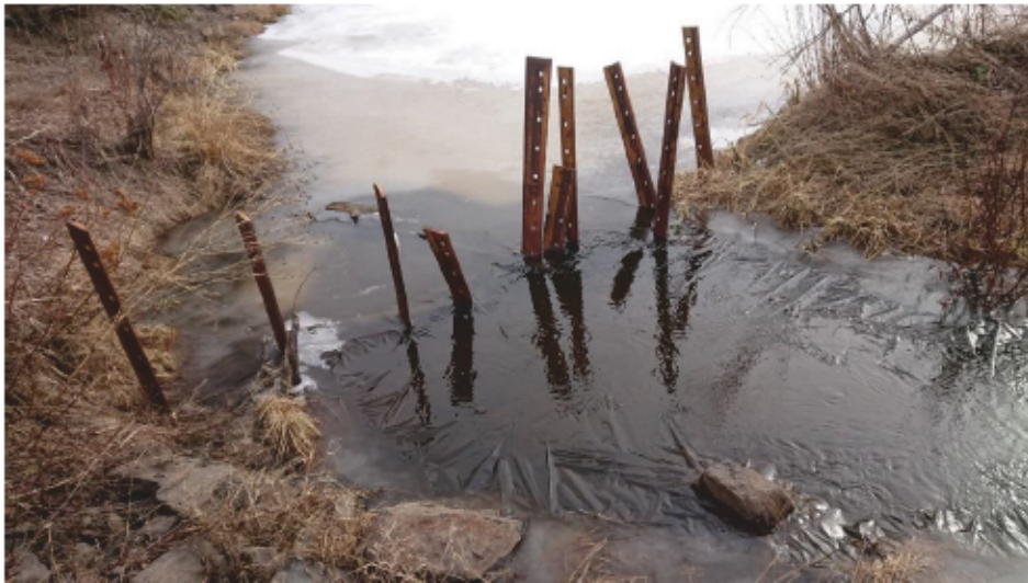
Figure 6-1 : Existing Debris Barrier at Main Culvert Crossing Inlet (Sta. 104+91)
