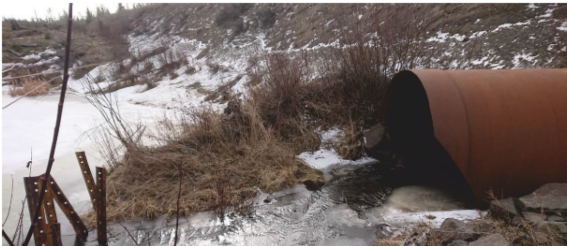
Figure 2-1: Existing 2400mm Steel Culvert Inlet in March 2021 (Main Culvert Crossing, Sta. 104+91)
