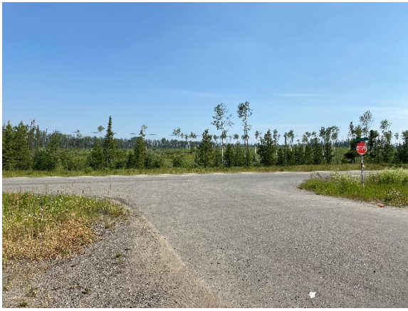
Photo 1: View north of the Shallow Bay Road intersection with Highway 16.
