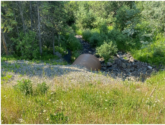
Photo 3: View downstream of the 2400 mm steel culvert.
