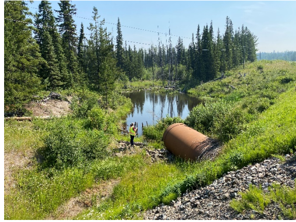
Photo 8: The pond immediately upstream, of the existing crossing, looking northeast.
