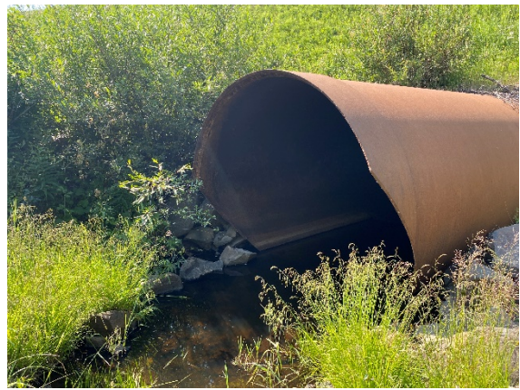
Photo 9: View of the 2400 mm steel culvert inlet from the pond.
