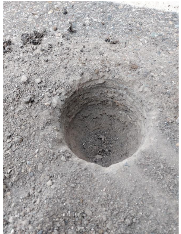
Photo 10 TH21-03 road structure
