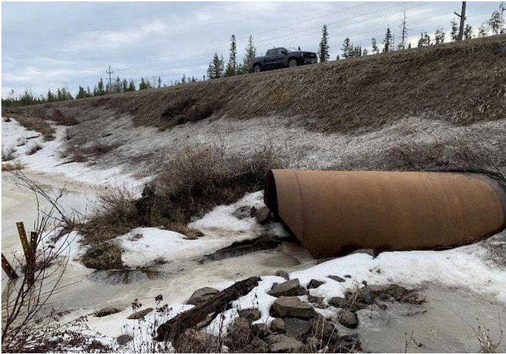
Photo 35 Culvert on the Northern Highway Side near STA 105+00
