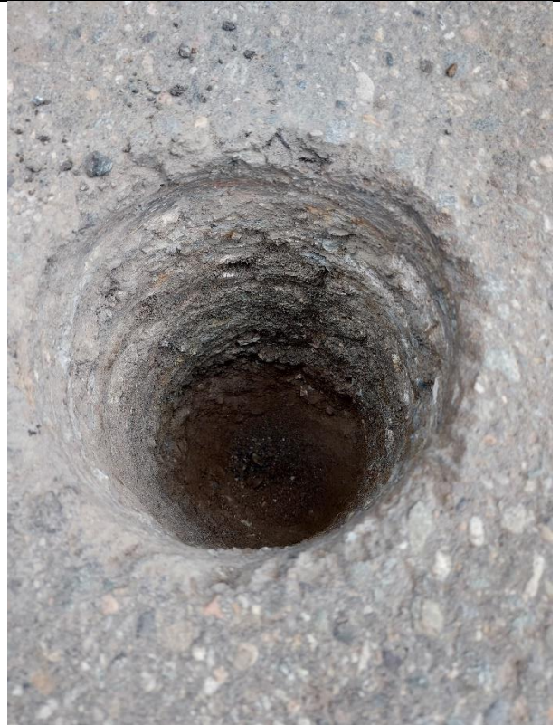
Photo 14 TH21-06 pavement structure drill hole
