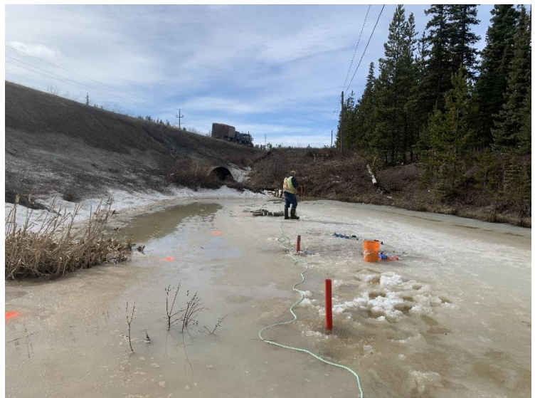
Photo 36 Excavation equipment used for test pits
