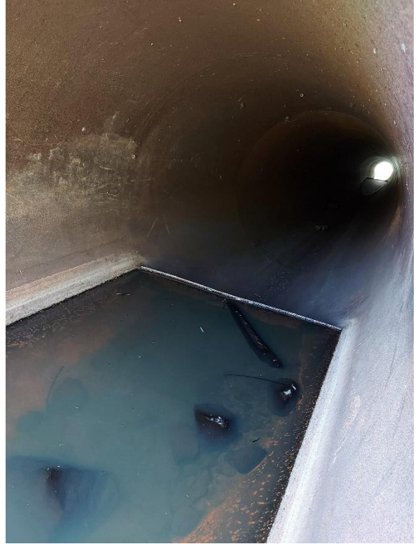
Photo 2 Existing culvert internal baffles
