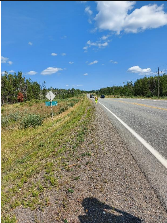
Photo 3 Facing west towards south embankment between Highway 16 and Frontage Rad
