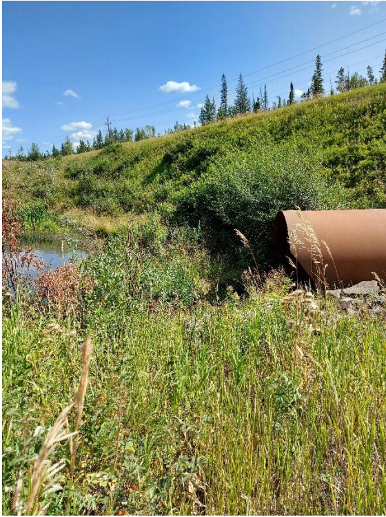
Photo 1 Facing east towards culvert inlet at northern embankment at Highway 16
