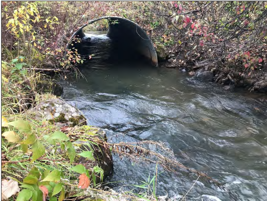
Figure 15: Outlet of Henry Road culvert looking upstream (McElhanney Sep. 30, 2020).
