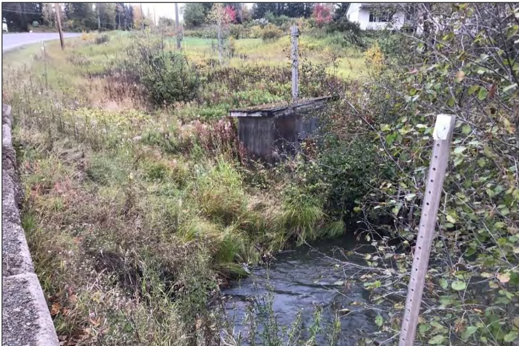
Figure 6: Kathlyn Creek III culvert outlet pool with old pumphouse to northeast.
