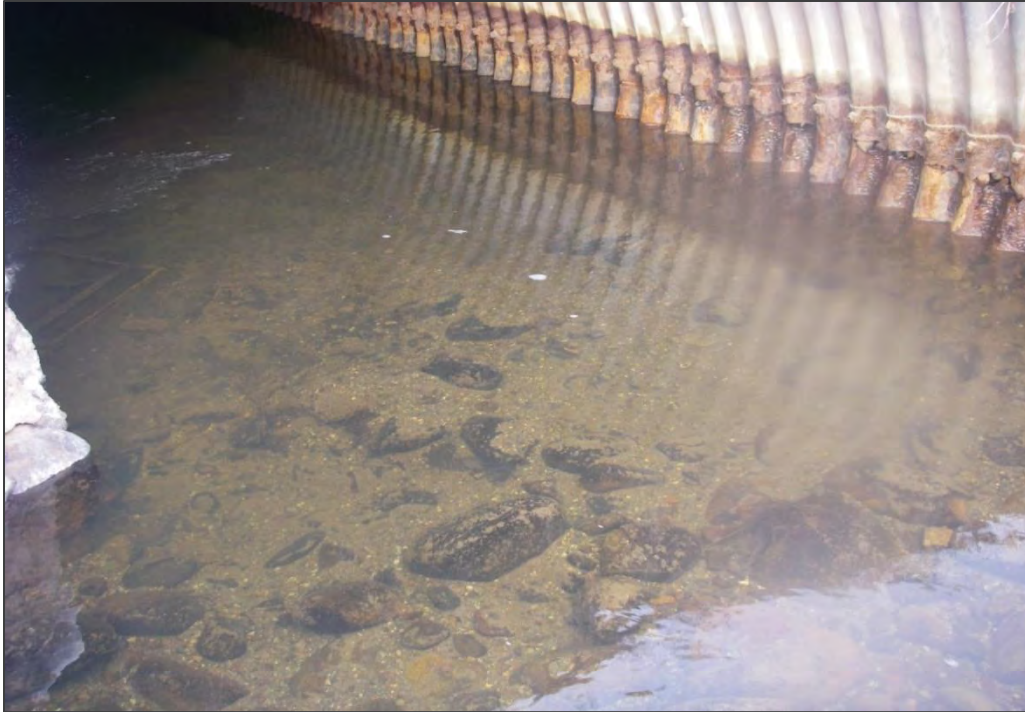
Figure 5: Kathlyn Creek III culvert outlet with naturally infilled bed material.
