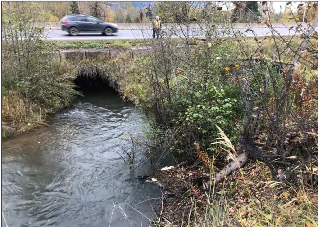
Figure 4: Kathlyn Creek III culvert outlet.
