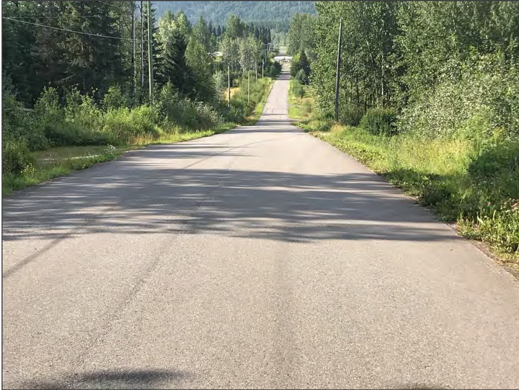
Figure 24: View south on Henry Road from crest of hill to the existing culvert on Kathlyn Creek.
