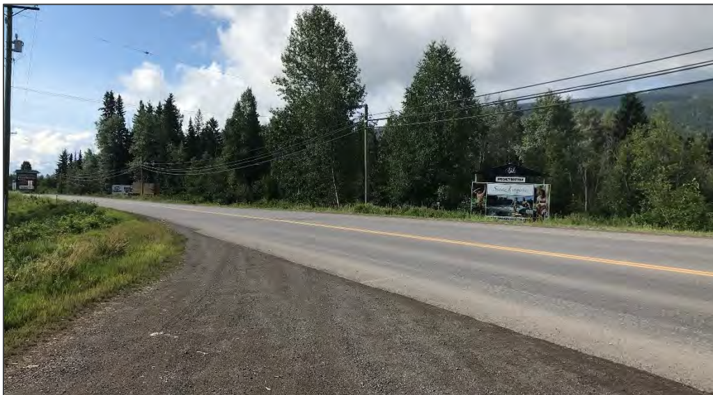
Figure 13: View southwest to proposed new intersection of Lake Kathlyn Road and Highway 16.
