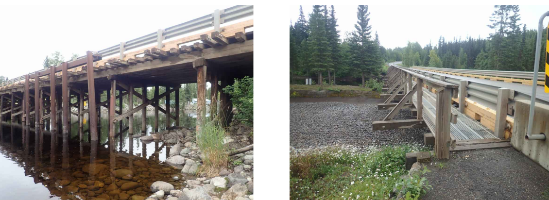
GENERAL CONTEXT OF EXISTING BRIDGE
