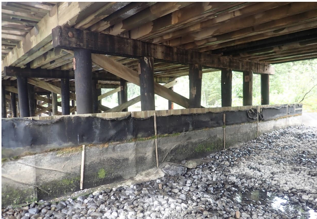
Photo 4: Spawning channel right bank, looking upstream. Vertical wood wall prevents berm overtopping into Fulton River (August 15, 2020).
