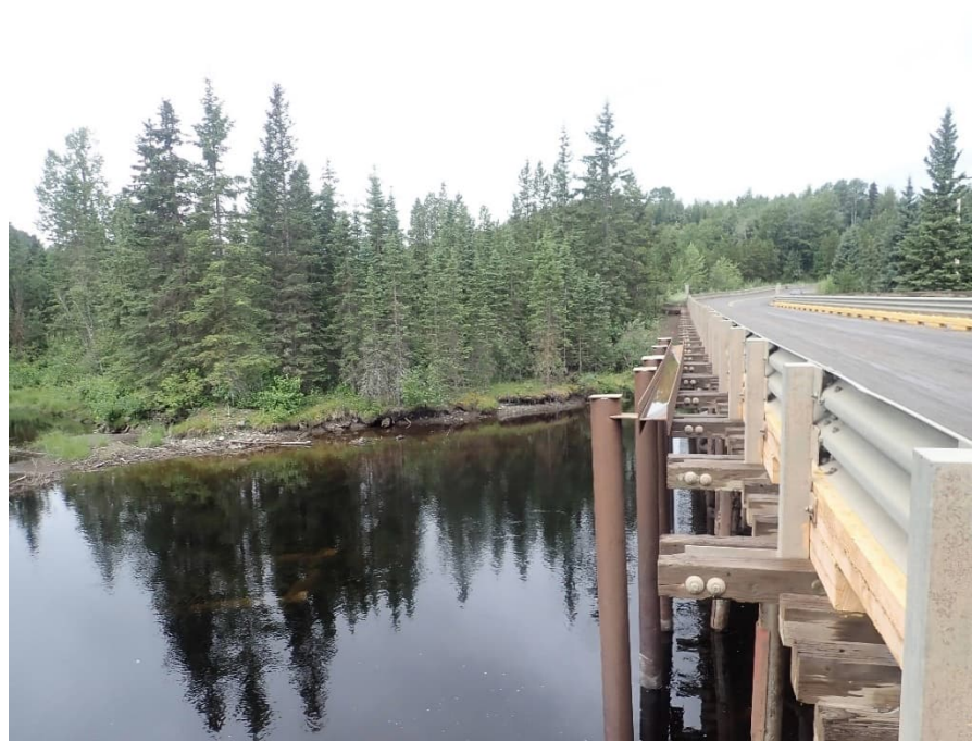
Photo 6: Fulton River crossing, left bank, looking upstream. Note the undermining of vegetation from erosion on the upstream bank (August 15, 2020).
