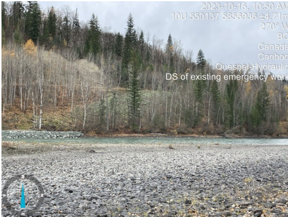
Photograph 1: View west across Quesnel River of proposed bank protection area, showing downstream end of previous (2023) rock placement and access path, 16 October 2023.
