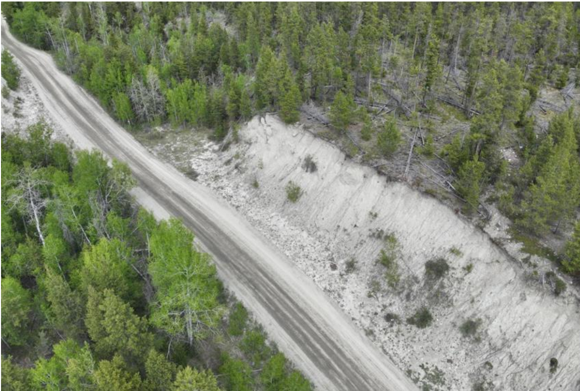
Drone photo taken from same location as previous photo, facing northeast.
