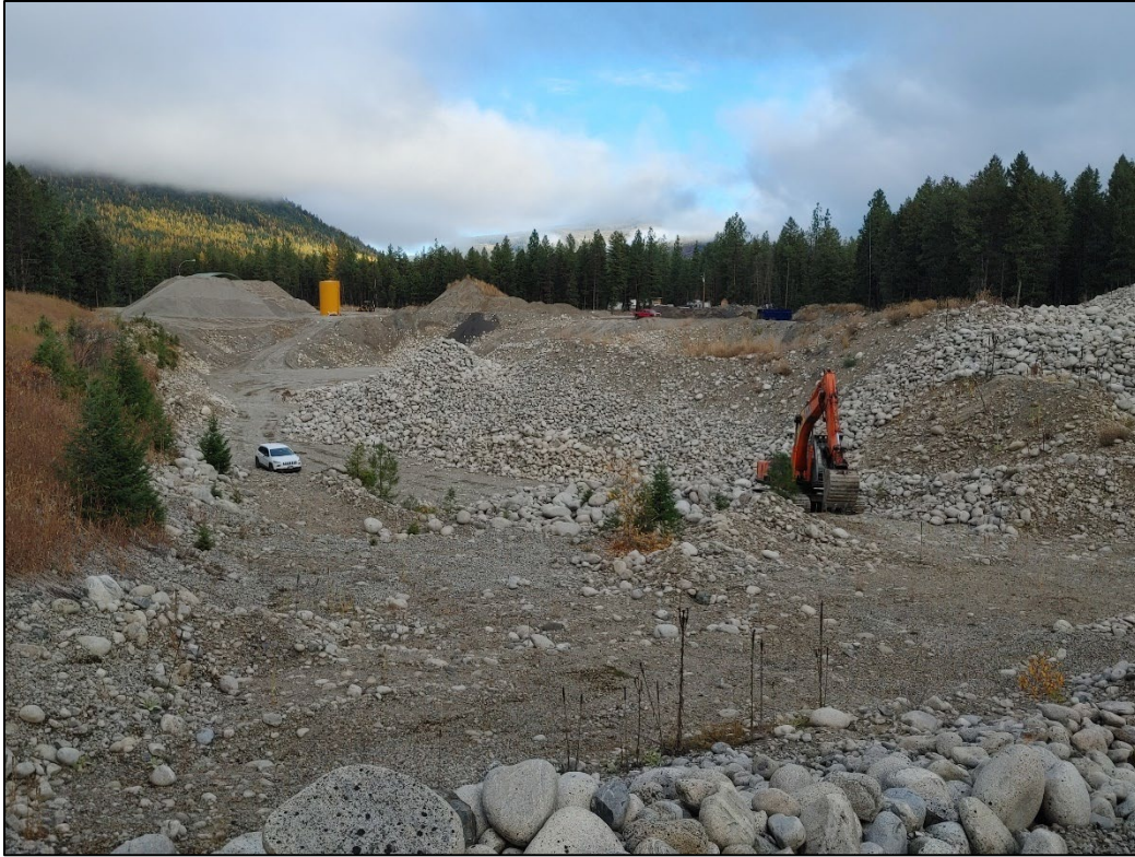
Photo 1 View from the top of the southern face looking north (October 2023).
