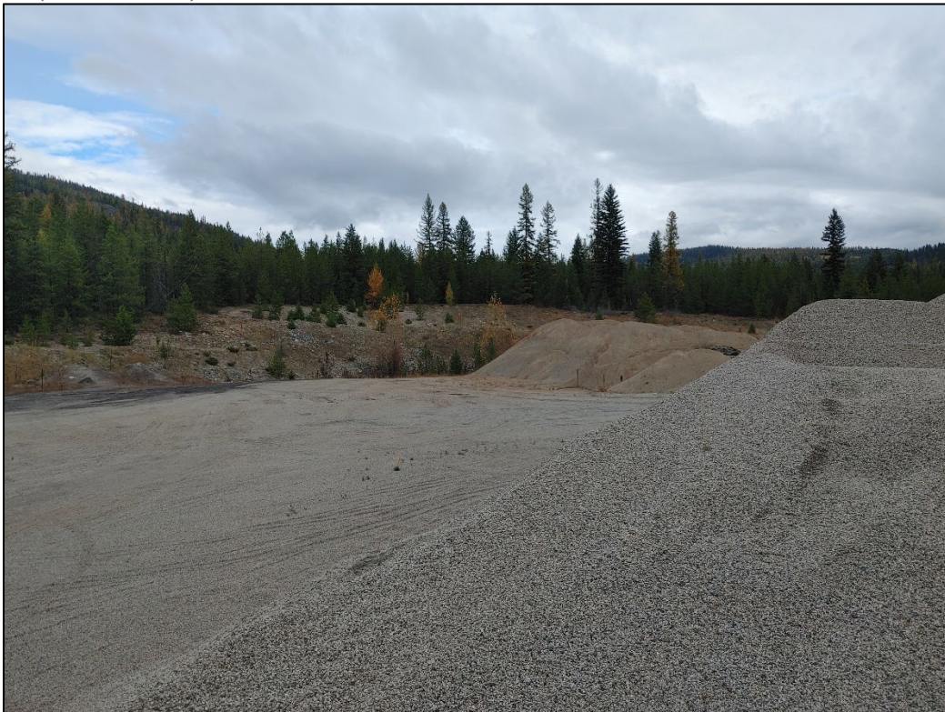
Photo 2 Proposed stockpile area in the northern part of the pit, looking north. Note stockpile of crushed aggregate and another near the face. (October 2023).
