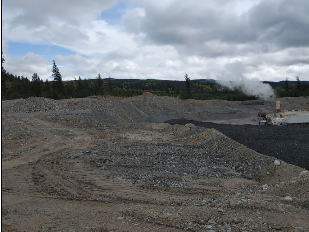
Photo 5 Top of pit face looking north. Note: the crusher and processed aggregate stockpile are no longer there (September 2023).
