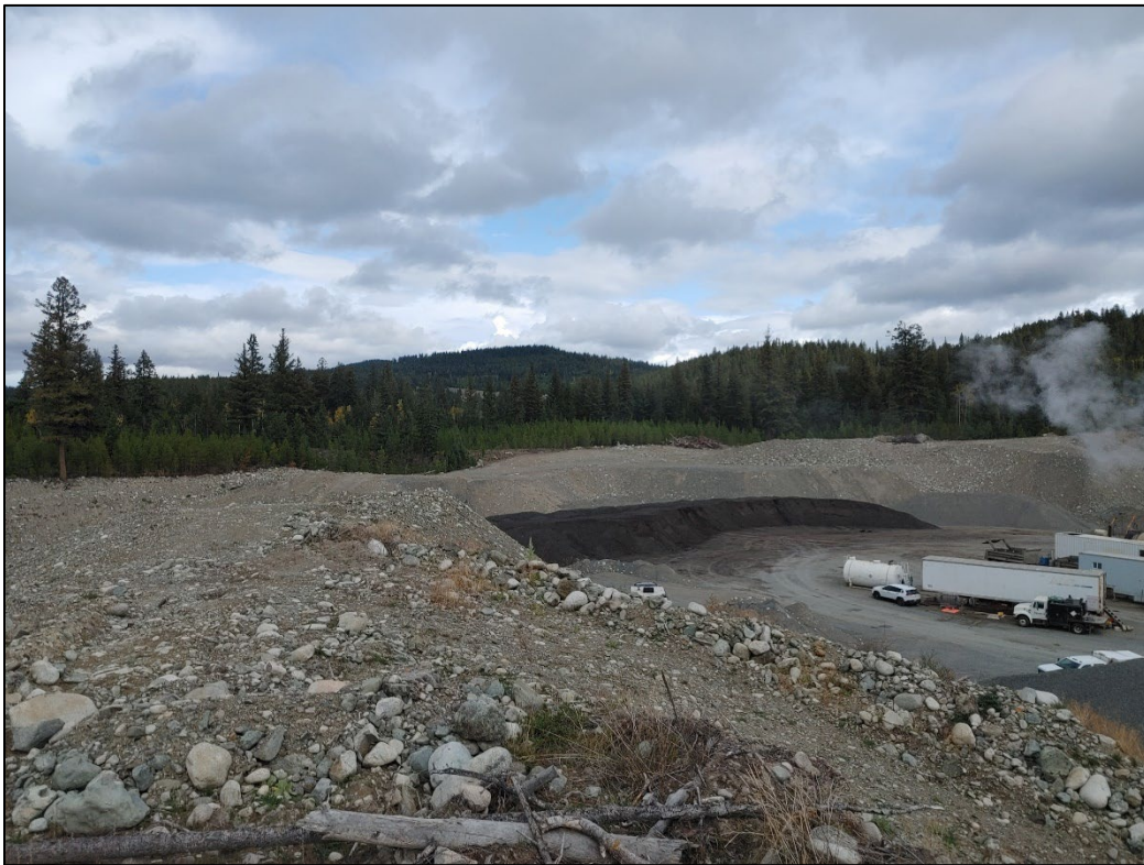
Photo 4 View from top of pit face, looking north at the pit face and crusher set-up area. Note: the crusher and processed aggregate piles are no longer there (September 2023).
