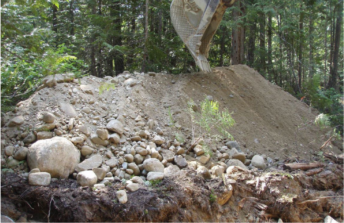
TP14-12 spoil material
