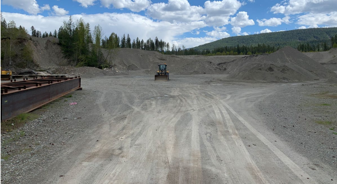
Facing south from the pit entrance. Stockpiles and material in this area of the pit may need to be relocated for stockpiling (May 2022).
