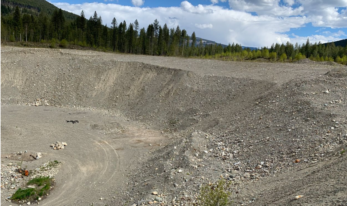
Facing southeast toward main pit face. Recommend crusher setup here (May 2022).
