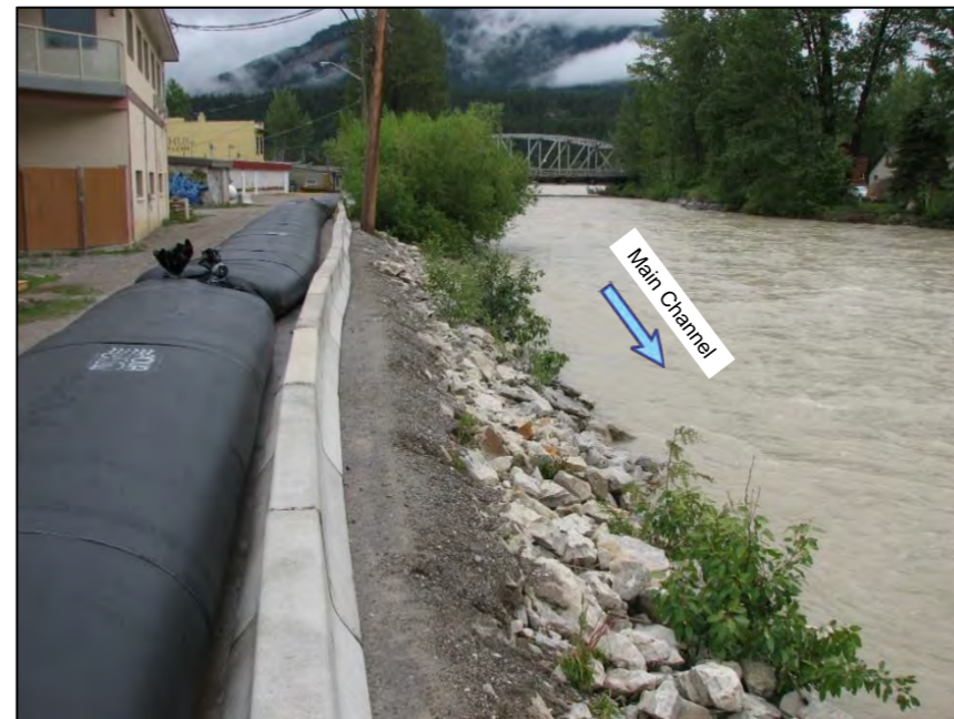
Bridge 1 visible in background. The Town of Golden installed rubber dams and jersey barriers to provide temporary additional dike freeboard during the June 2012 flood. Photo taken by the Town of Golden on June 7, 2012.
