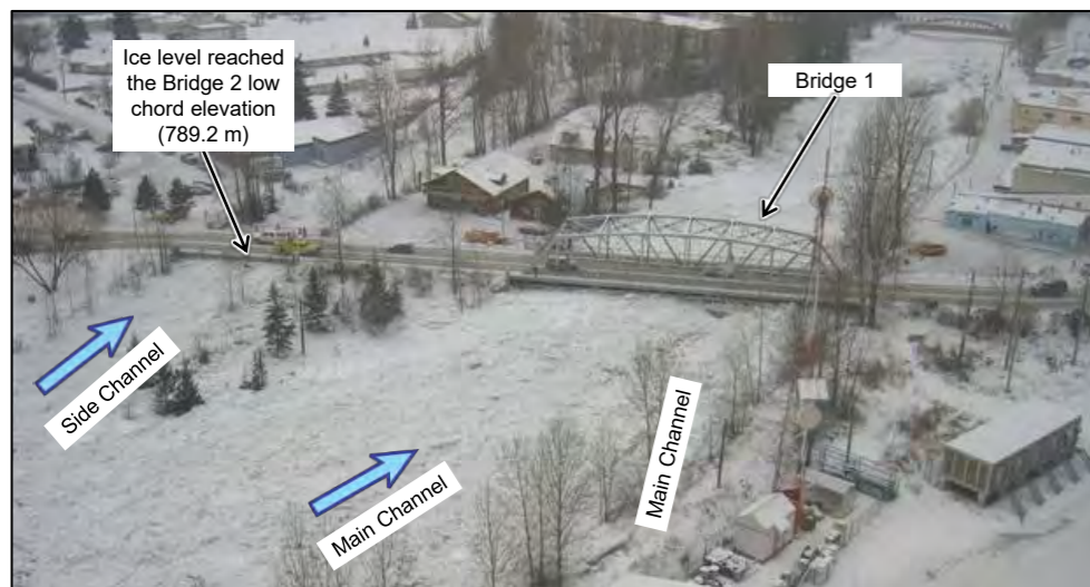
View of the Highway 95 bridges from a helicopter reconnaissance. Photo by Paul Doyle, P.Eng. of BC Rivers Consulting (formerly of BC of Ministry of Forests Lands and Resource Development) taken on December 20, 2005 (the same day as the peak of the ice jam).
