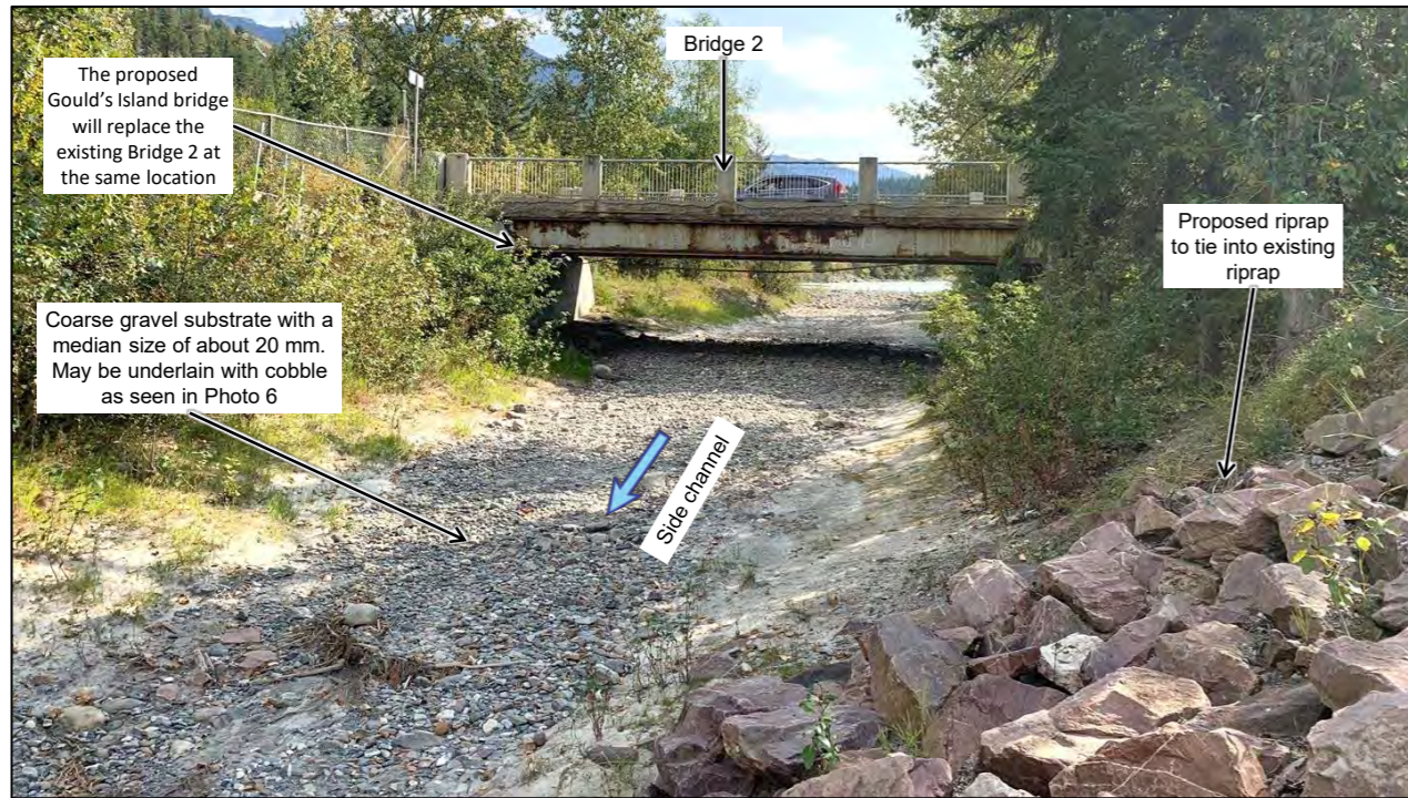
Photo 5: Downstream of Bridge 2. Photo taken on October 22, 2020 by Stantec.
