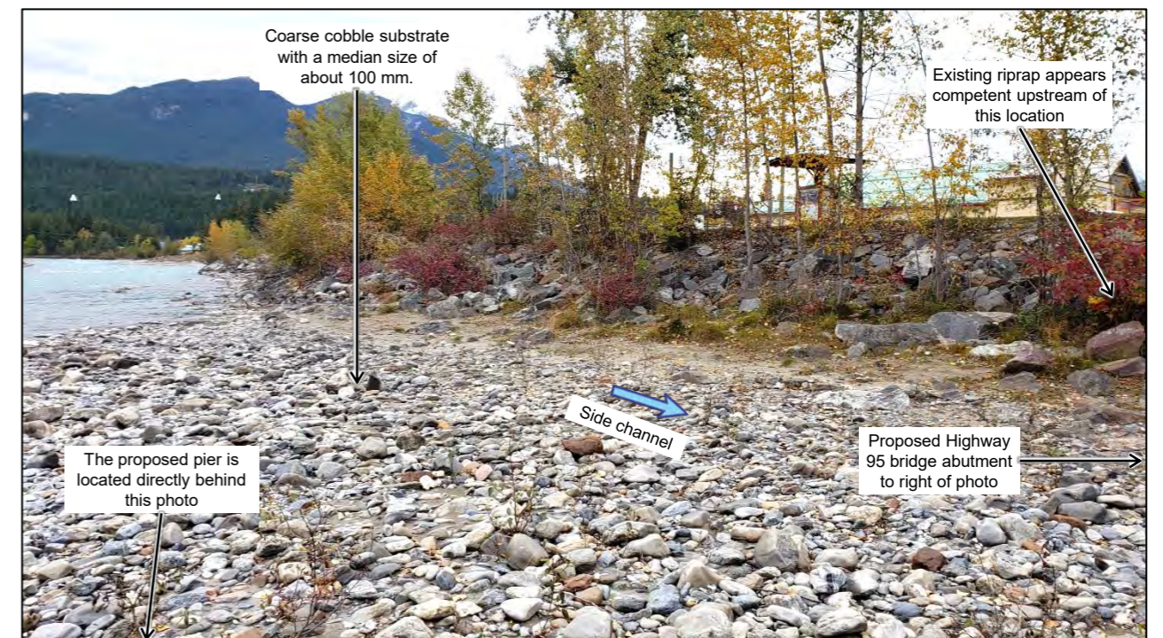
Photo 8: Left (south) bank upstream of proposed Highway 95 bridge abutment. Photo taken on September 29, 2019 by Matrix Solutions Inc.
