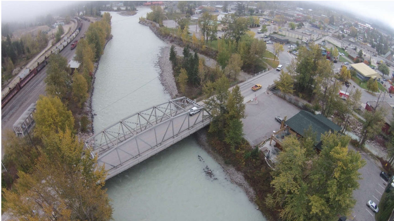
Figure 2. Aerial view of existing Kicking Horse River Bridges 1 and 2
