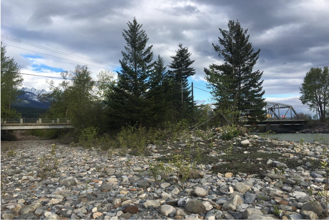
Photograph 19: Section 6 and 7 – Looking west, downstream at Substrate of Kicking Horse River main and side channel.
