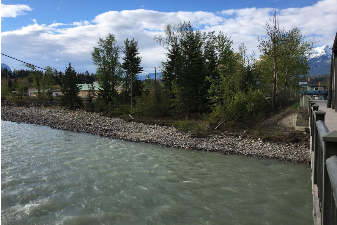
Photograph 15: Section 7 – Looking south, vegetation of median.
