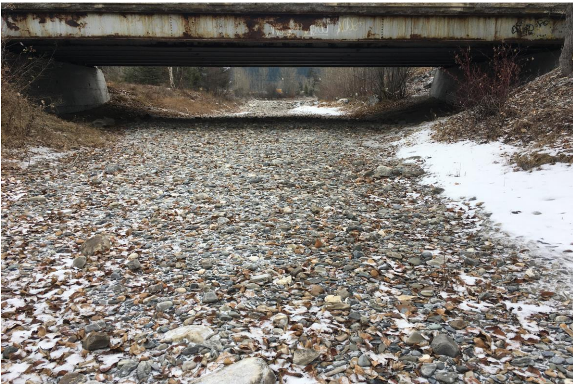
Photograph 8: : Section 3/4 – Looking east, upstream at Substrate of side channel.
