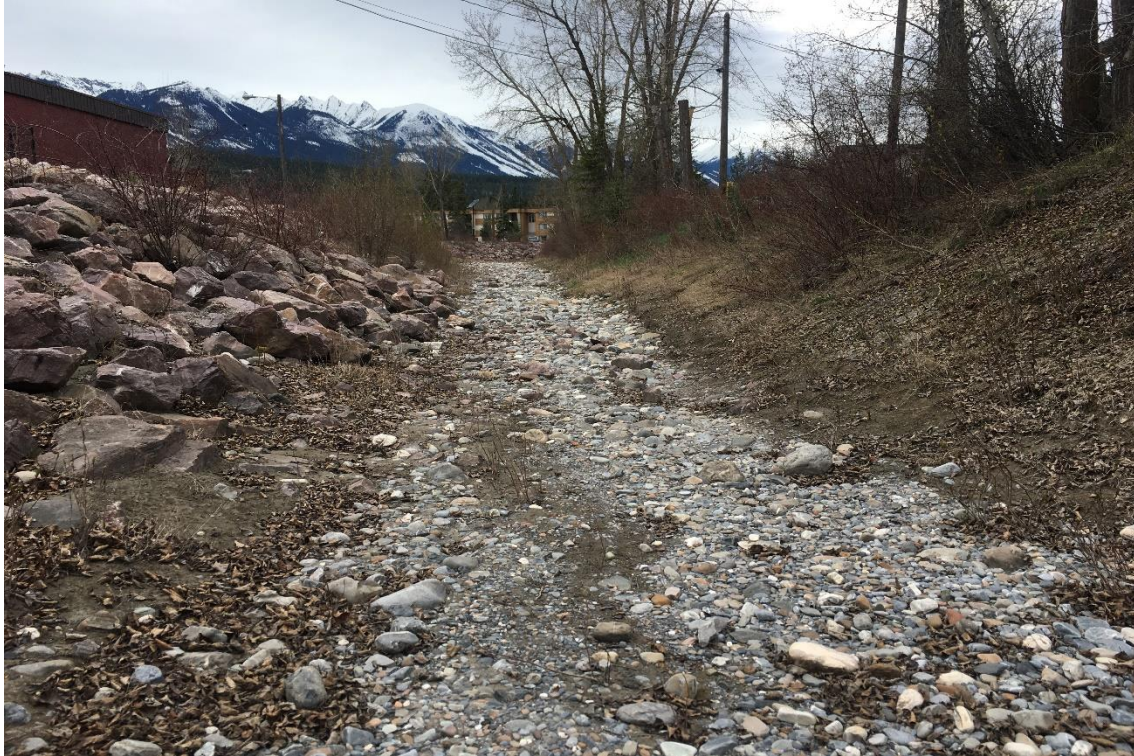
Photograph 7: Section 3 and 4 – Looking west, downstream at Substrate of side channel.
