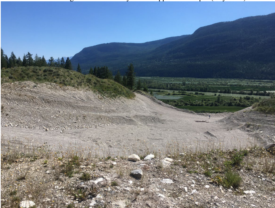
View looking south from edge of developed pit face onto crusher floor setup area, upper floor (July 2018)
