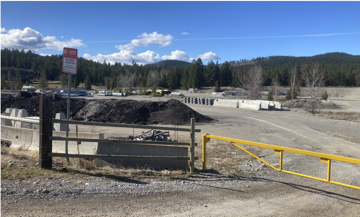
Facing south from pit entrance toward Area B. Materials stored in this area will have to be relocated prior to future mining in this area. (April 2022).
