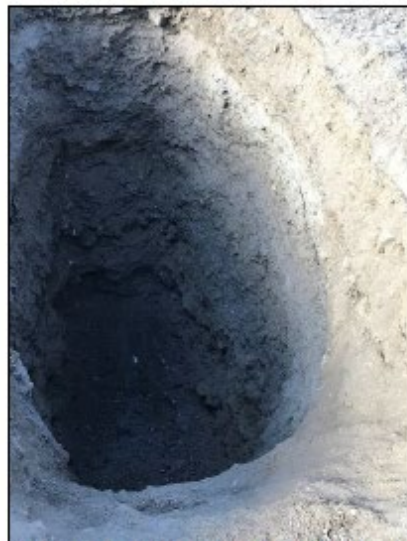
Test Pit 18-07 (gravel to 5.0 metres)
