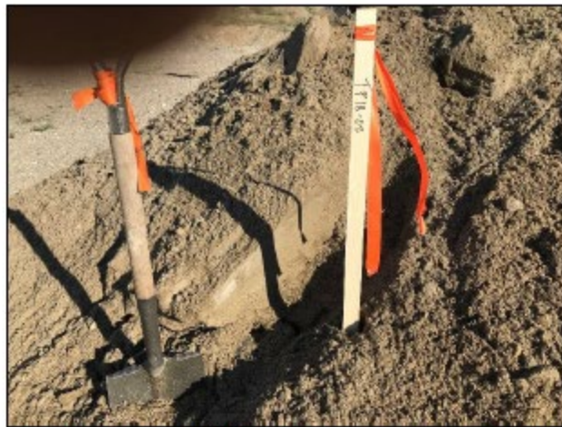
Test Pit 18-02 Spoil (SM 3 between shovel and stake)
