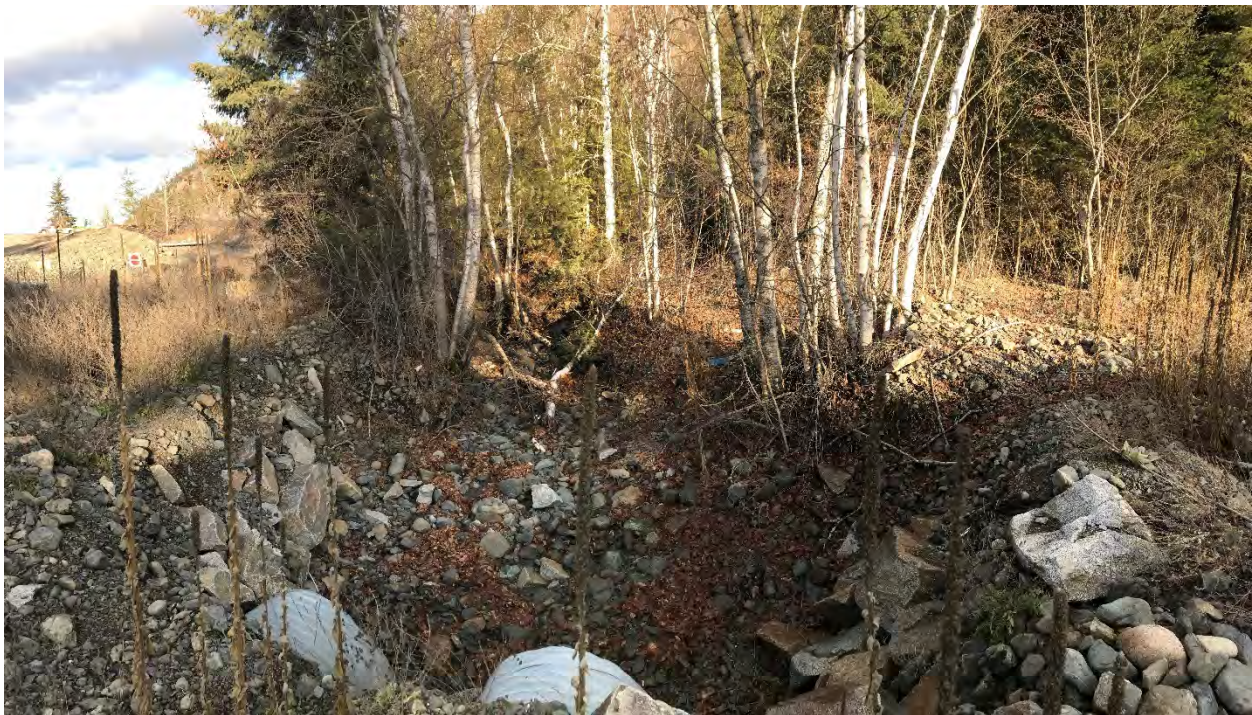
Figure 2-8. Upstream view of Skwootum Creek at Dunn Lake Road. BGC photograph of November 28, 2018.
