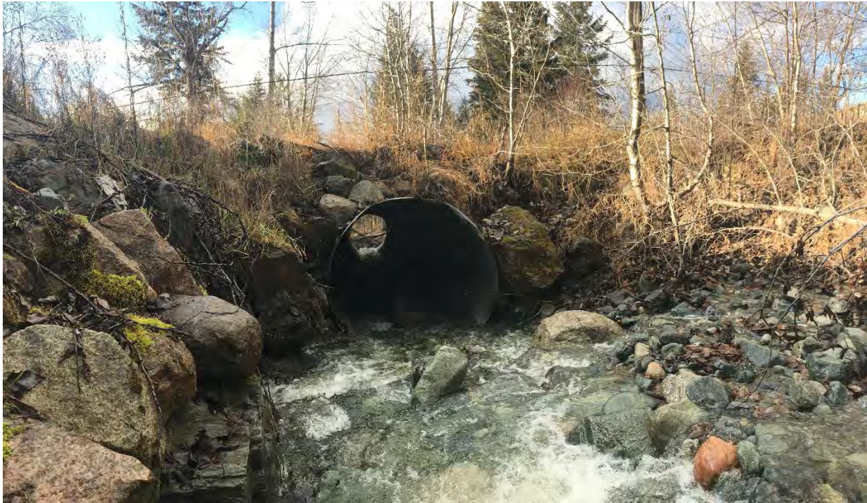
Figure 2-4. Downstream view of 1.8 m diameter CSP culvert inlet on Newhykulston Creek at Dunn Lake Road. BGC photograph of November 28, 2018.
