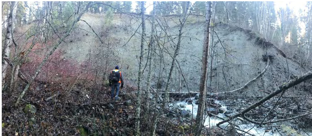
Figure 3-4. Unstable valley slope on south side of Newhykulston Creek (site WP 6, Drawing 03). BGC photograph of November 28, 2018.
