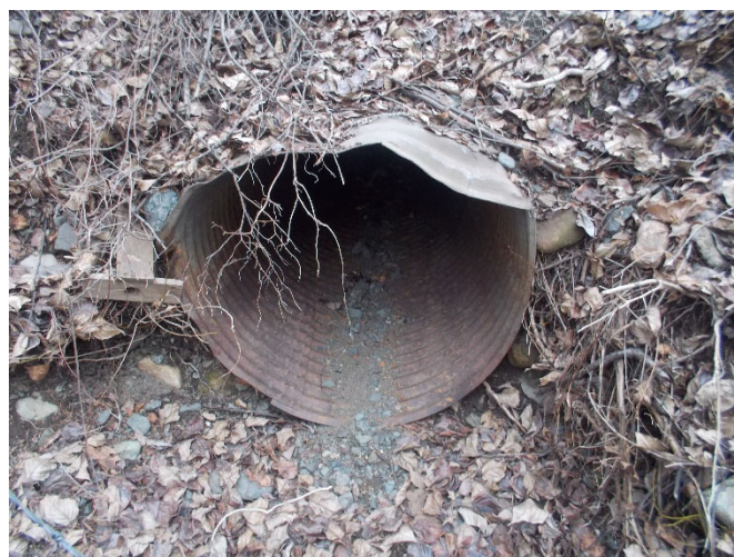
Photo 4. Skowootum creek - 1000mm culvert outlet at CN ROW
