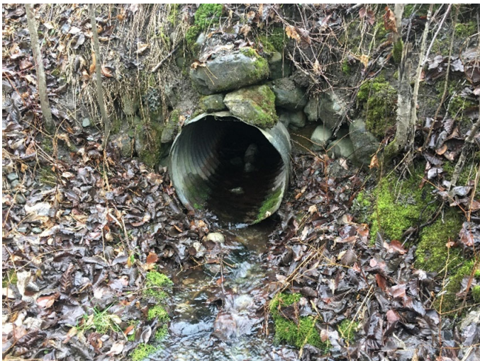
Photo 11. Kikwilli creek - 600mm CSP at outlet
