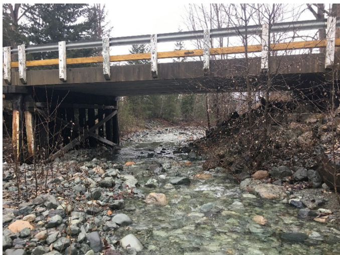
Photo 17. Chu-Chua creek - Dunn Lake Road bridge crossing
