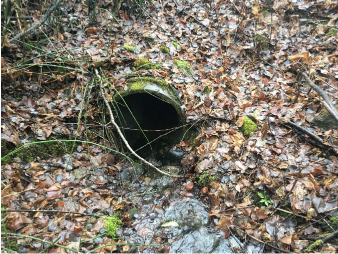
Photo 9. Kikwilli creek - 600mm NCSP at inlet
