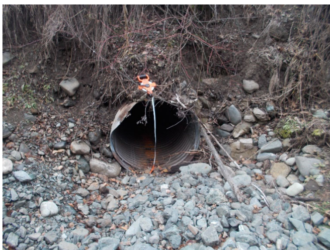
Photo 3. Skowootum creek - 1000mm culvert inlet at CN ROW
