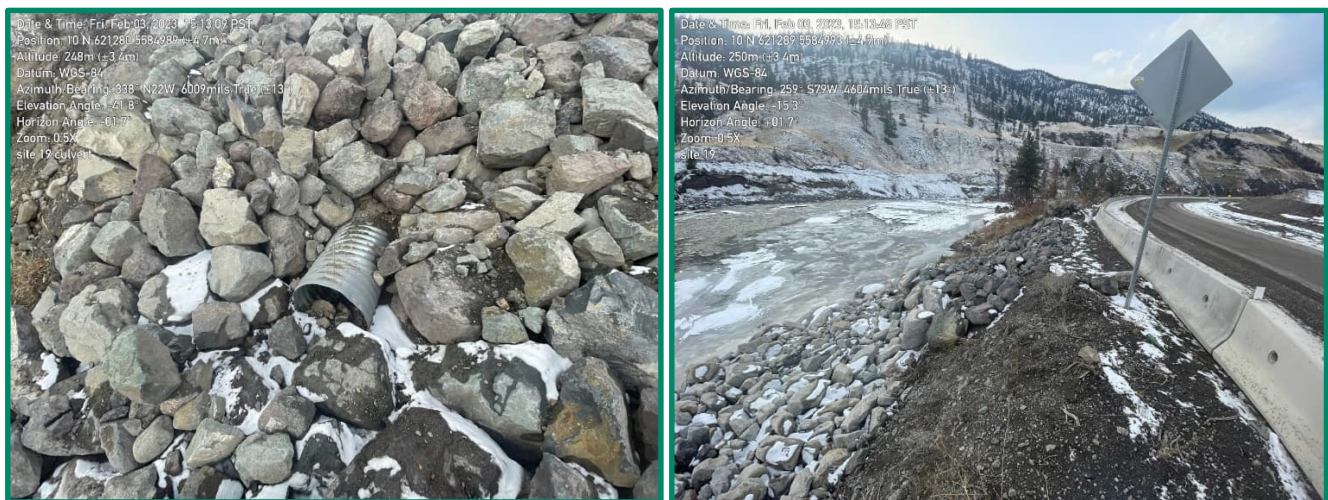
Figure 2.7 Site 19 Existing 600mm CSP culvert
