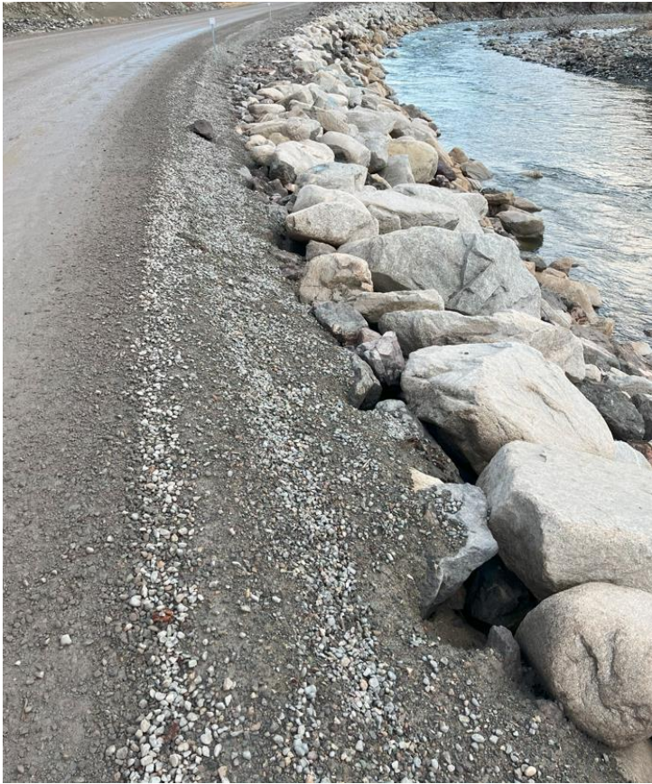
Photo: Site 19 view upstream illustrating transition in granular filter.
