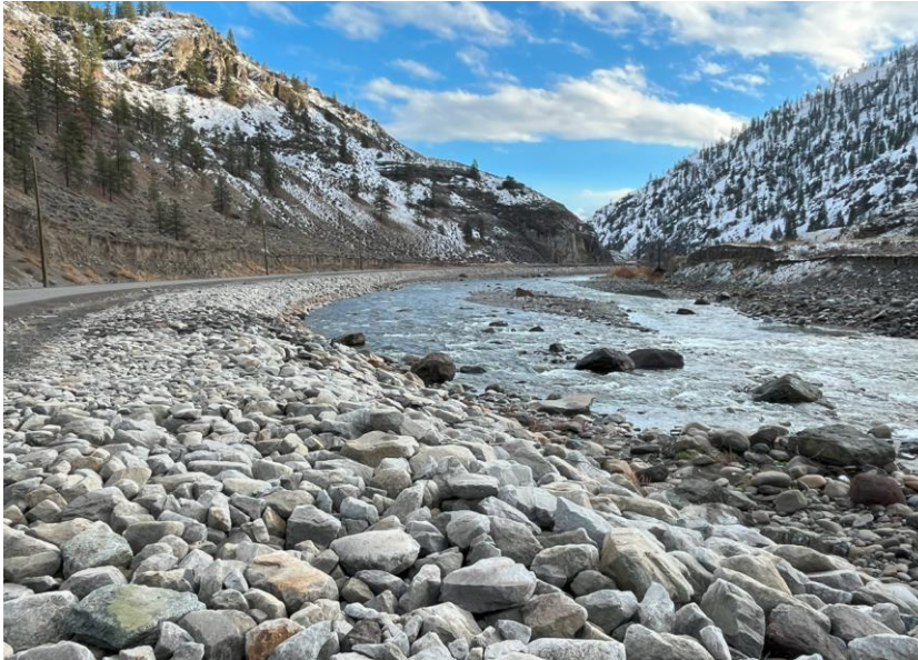
Photo: Site 18 view upstream illustrating riprap voids and uphill slopes from the event.
