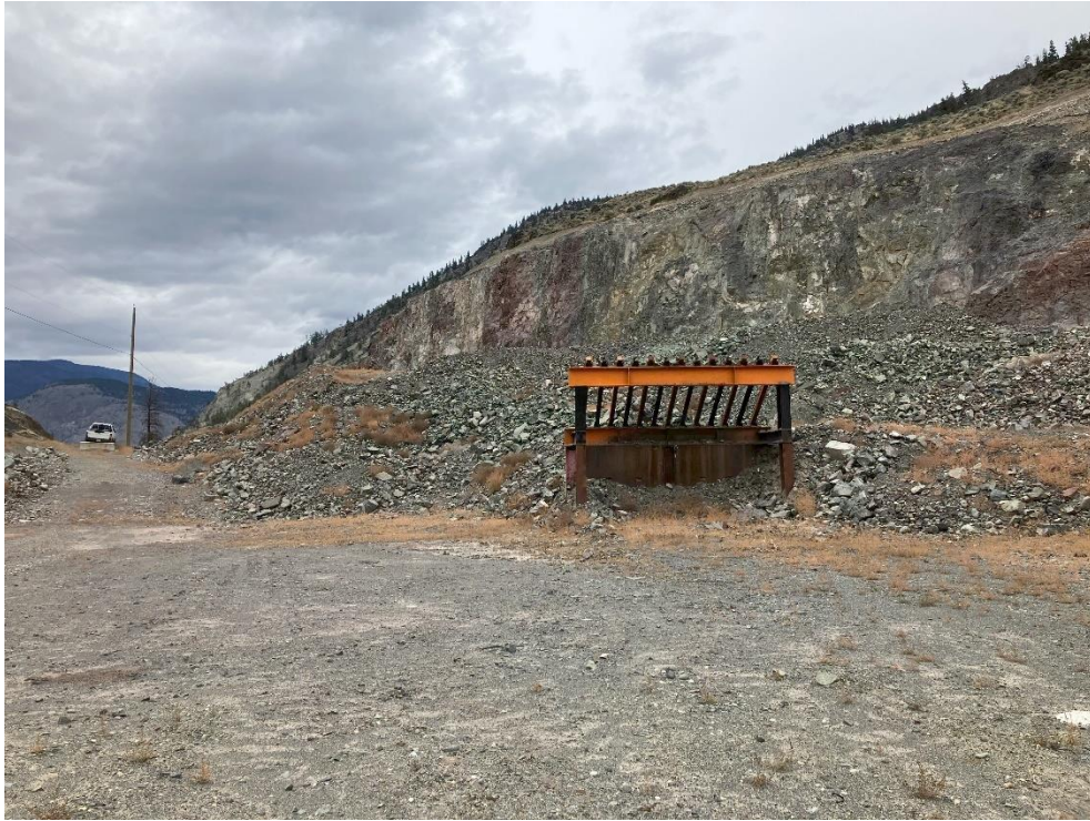
Photo 9. Stockpile of blasted rock at base of blasted face at Site 17 and grizzly, looking north.
