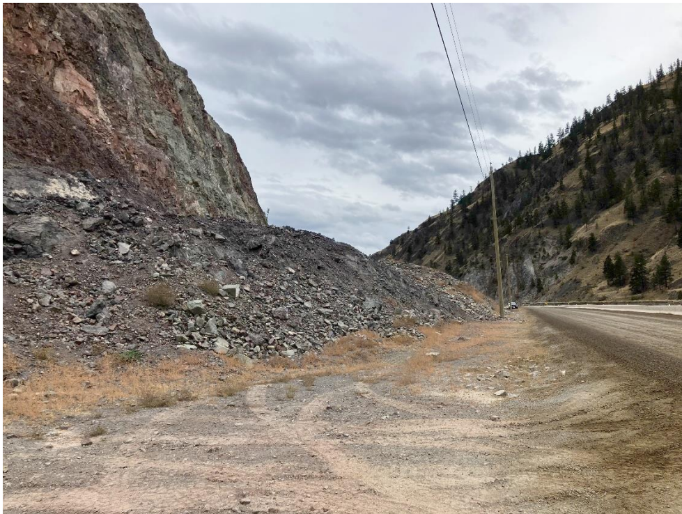
Photo 8. Stockpile of blasted rock at base of blasted face at Site 17, looking southeast from northernmost end.
