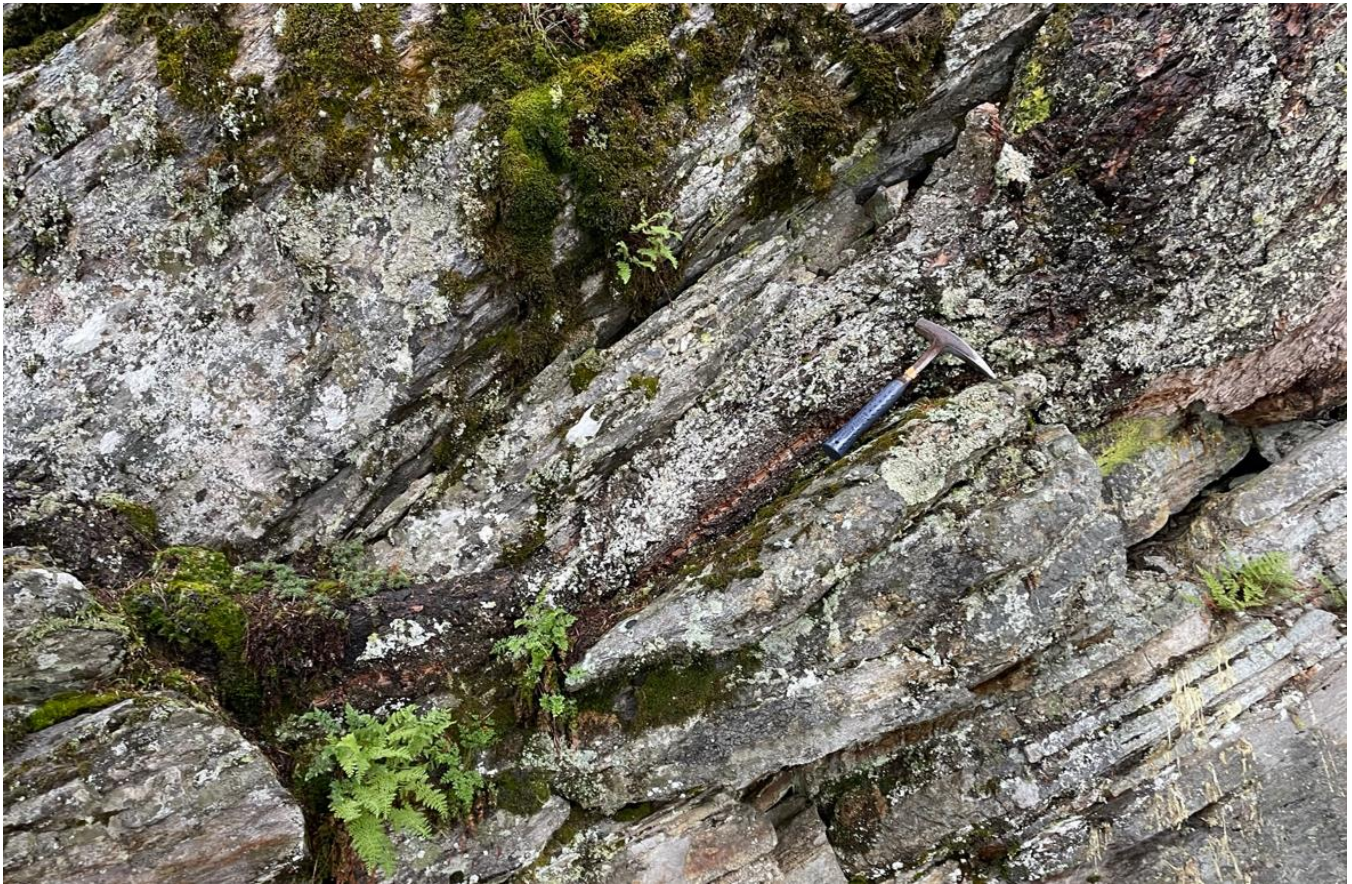
Photo 4 Rock Mass Immediately Upslope of Preferred Tower Location.
