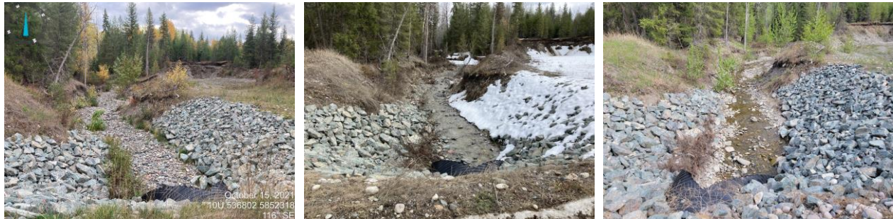
Figure 13 – View upstream; left photo October 2021, center photo March 2022, right photo May 2023
