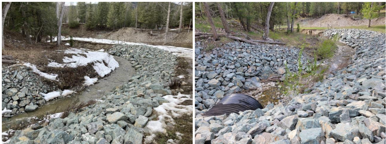
Figure 14 – View downstream; left photo March 2022, right photo May 2023
