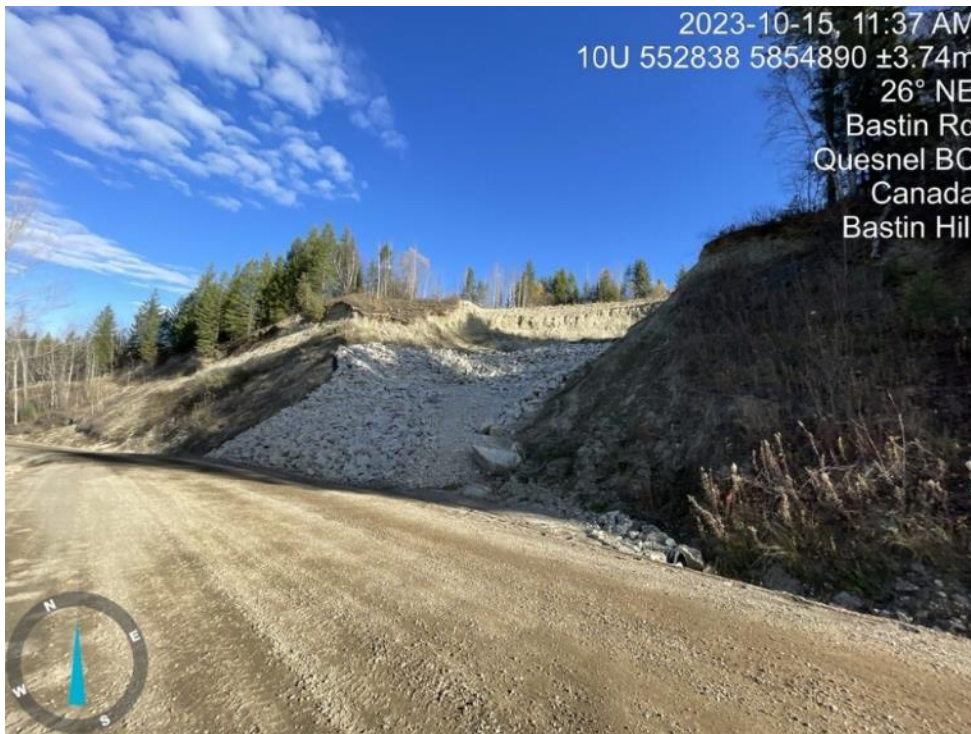
Photograph 7: Current slide condition at Bastin Road, showing mature trees on top of slope, 15 October 2023.
