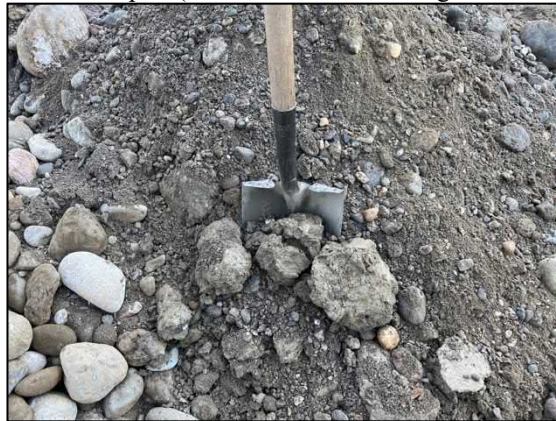
Test Pit 23-19 Spoil (Silt and clay mixed with gravel 5.0-5.5m)
