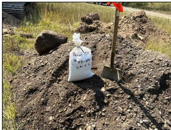
Test Pit 23-24 Spoil (Clean, coarse sand and gravel 0.9-5.5m)
