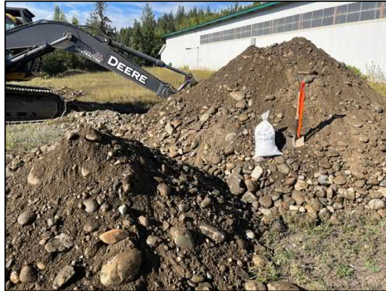
Test Pit 23-06 Spoil (Clean coarse sand and gravel 0.1-4.2m)
