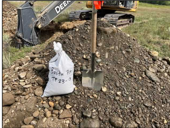
Test Pit 23-13 Spoil (Clean, coarse sand and gravel 0.1-5.5m)
