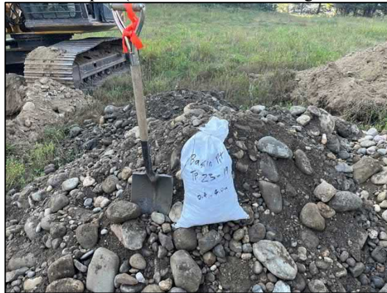
Test Pit 23-19 Spoil (Clean, coarse sand and gravel 0.4-5.0m)
