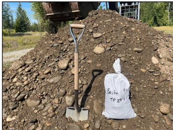
Test Pit 23-01 Spoil (Clean, coarse sand and gravel 1.5-5.2m)
