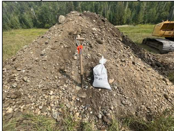
Test Pit 23-12 Spoil (Clean, coarse sand and gravel 0.4-4.0m)
