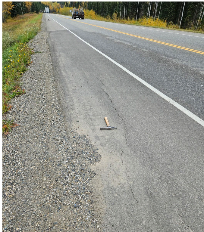
Photo 2 Cracks in pavement adjacent to the landslide headscarp, looking north, Sept. 25, 2023.
