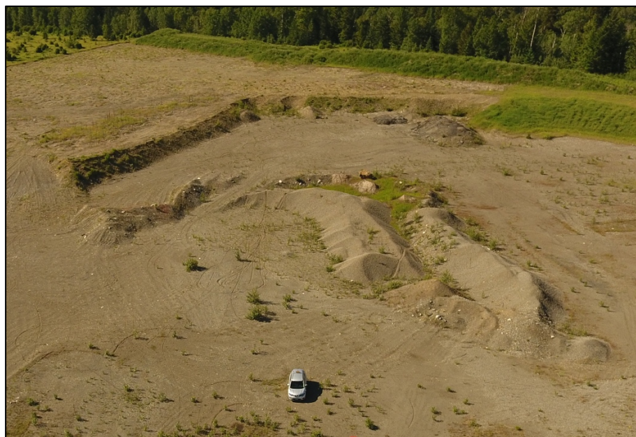
March 2015 Stripped Area Looking South
