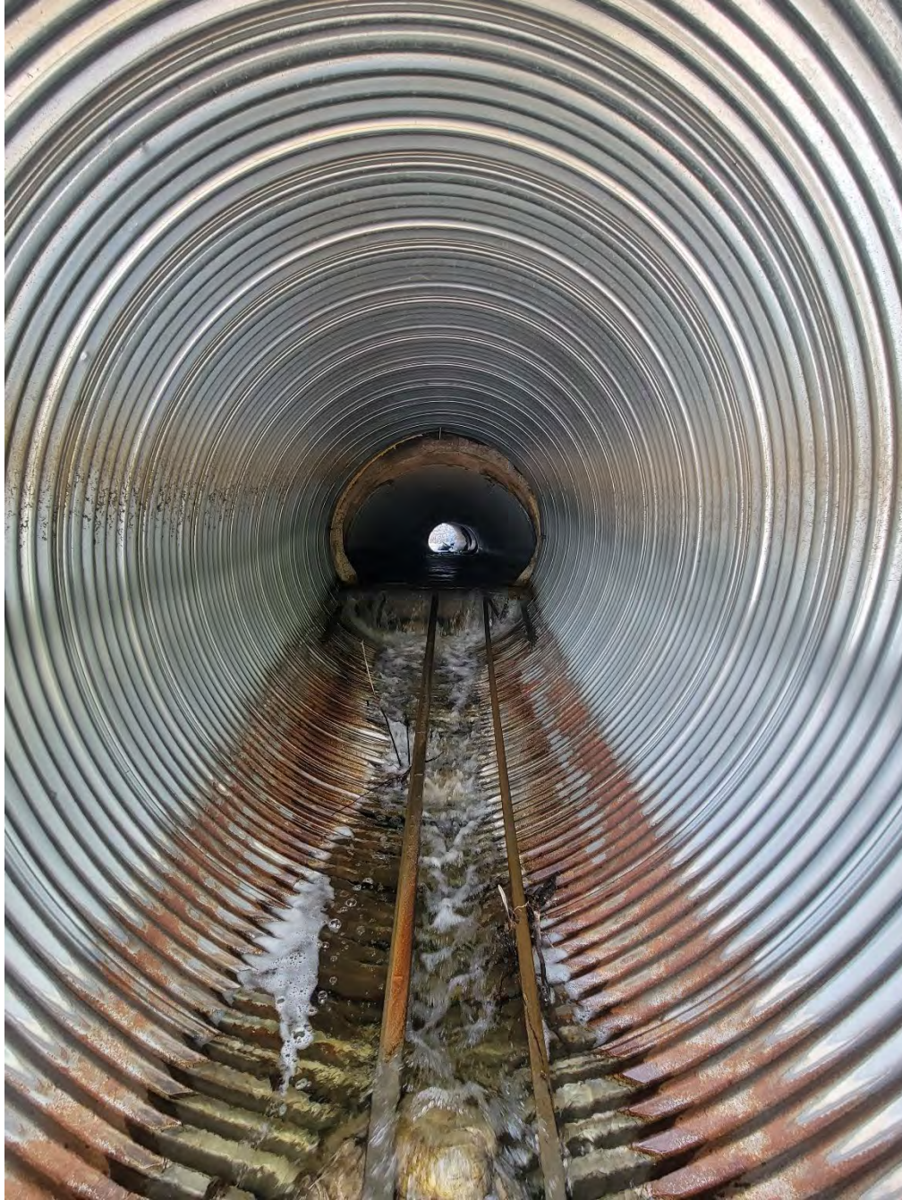
Highway 97 culvert facing upstream-northeast.
