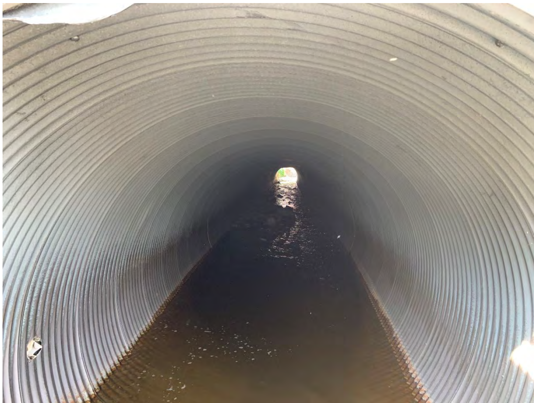
Reach 2 Site 1 Cache Creek Inn culvert – facing downstream.
