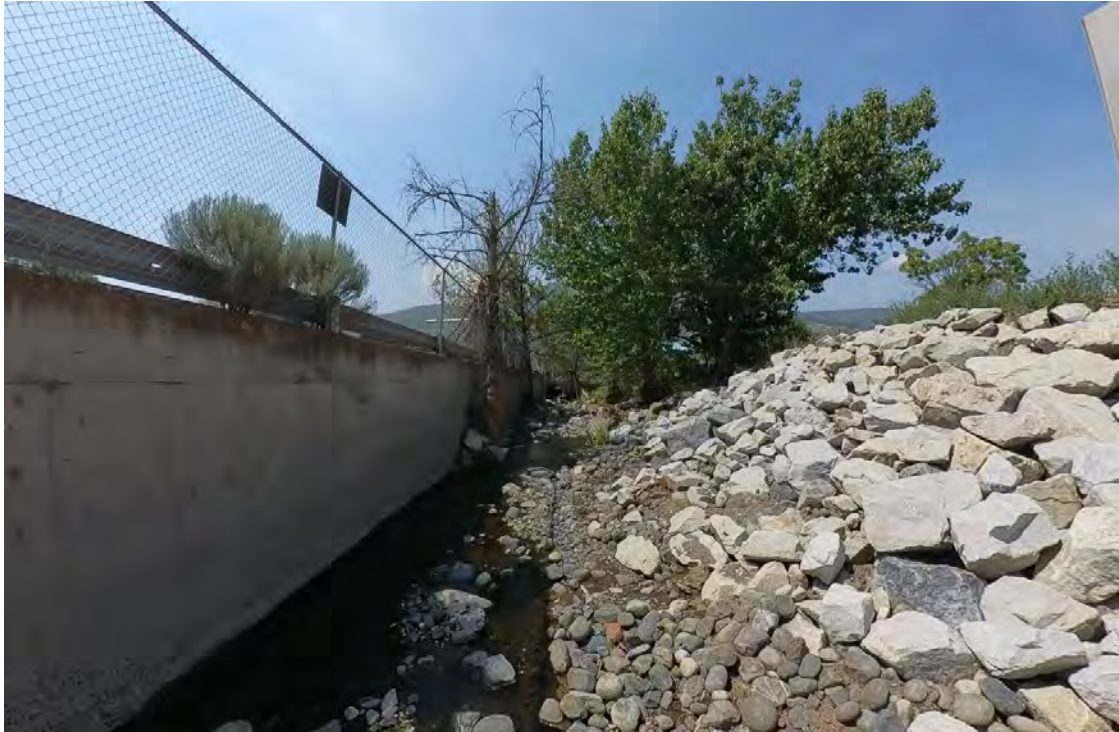
Reach 2 Site 1 upstream end of the site facing downstream.
