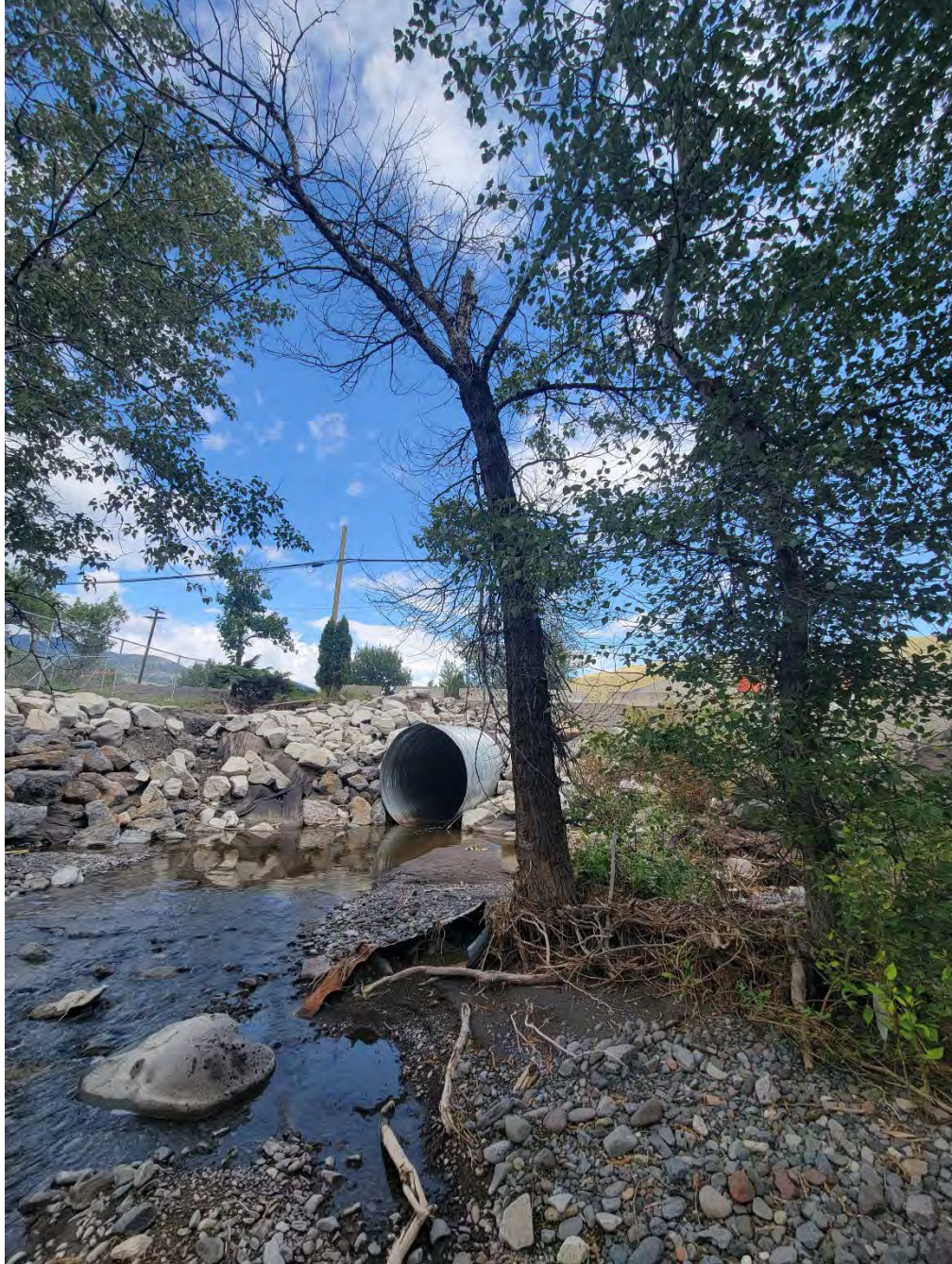
Highway 97 culvert and Reach 1 Site 2 deep pool-facing northeast.
