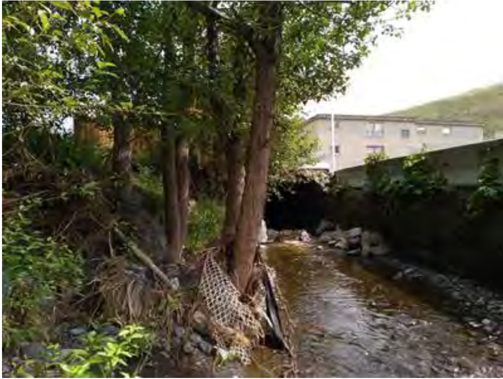
Reach 1 Site 1 cottonwood bunch 5 – to be removed.
