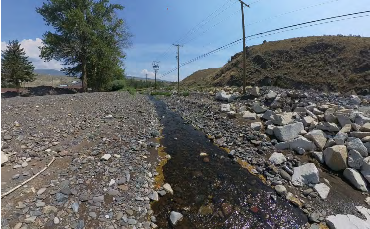
Reach 2 Site 2 upstream end of site.
