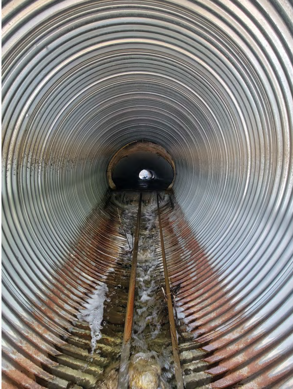
Highway 97 culvert facing upstream-northeast.
