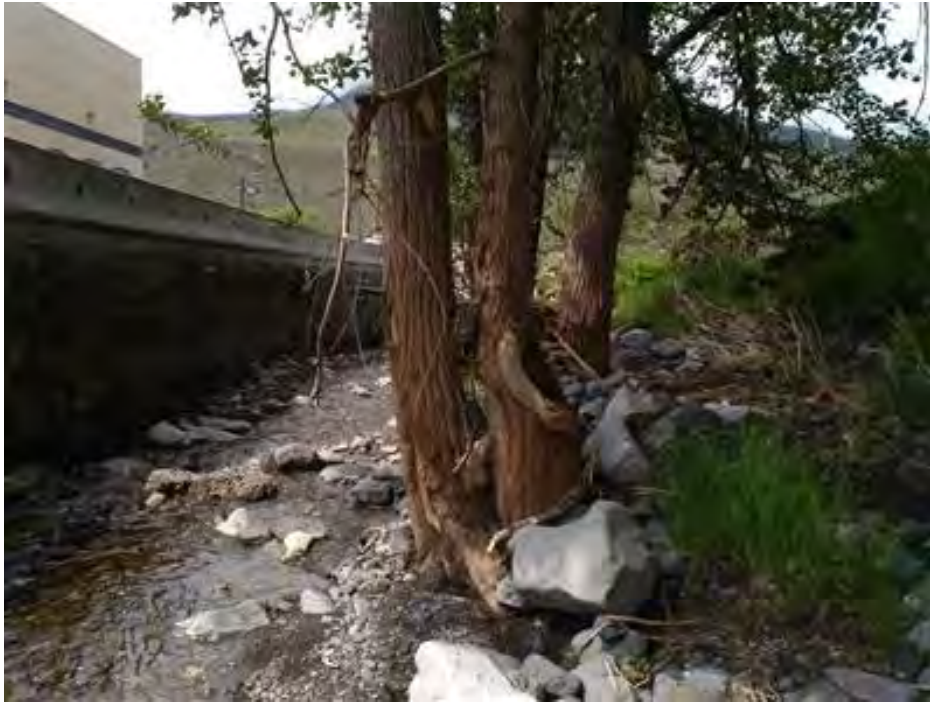
Reach 1 Site 1 cottonwood bunch 3 - to be removed.
