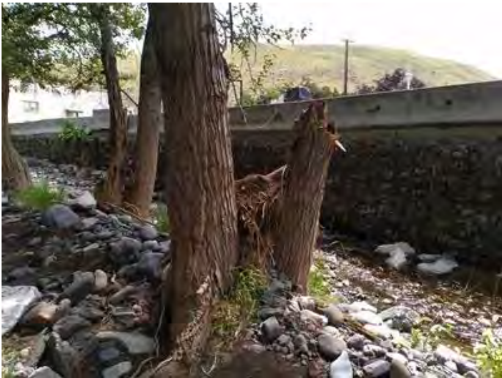
Reach 1 Site 1 cottonwood bunch 2 – to be removed.
