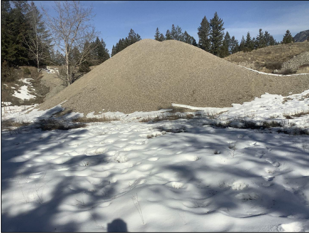
Figure 7 Stockpile 2. Available to use, it is recommended that the material be tested to determine the gradation and if it meets specifications (March 2023).
