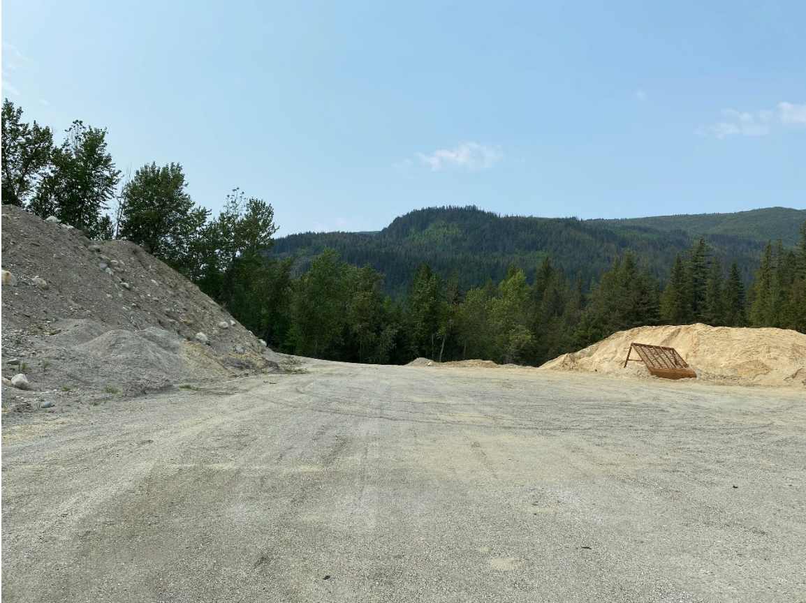
Crusher set up area, lower floor looking northwest, May 2023.
