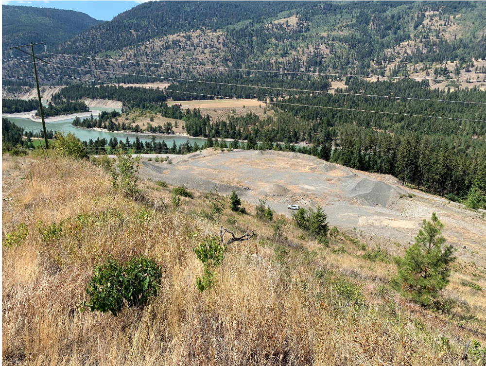
Looking down from suitability area onto proposed crusher set up site, facing southwest, August 2023.
