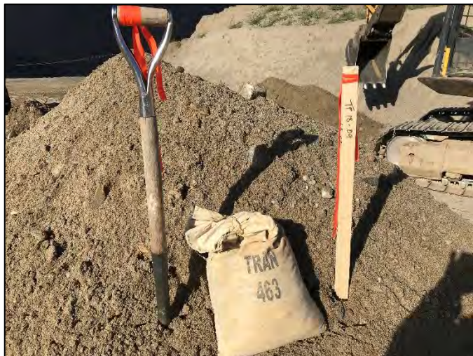
Test Pit 18-04 Spoil (0.0 to 3.1 metres)
