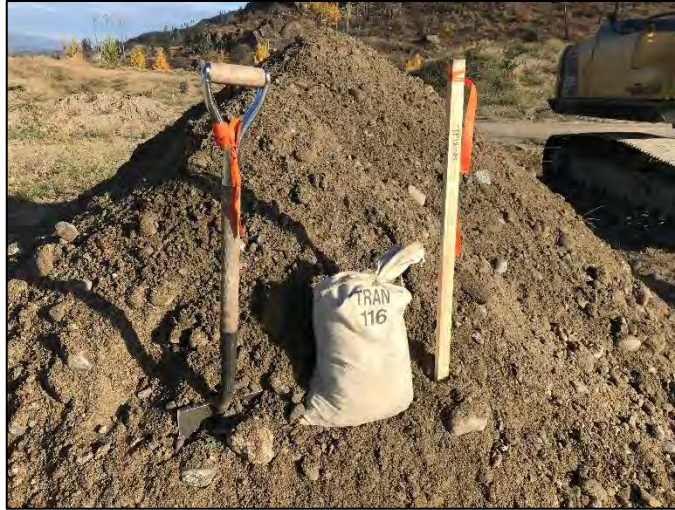
Test Pit 18-03 Spoil (0.0 to 5.0 metres)
