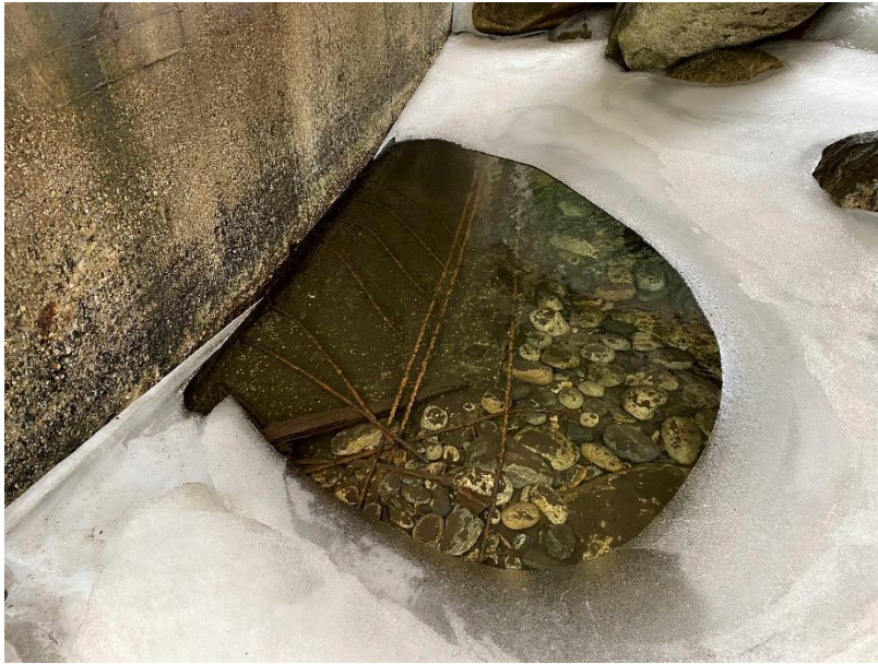
Photograph 1 Exposed rebar at the base of the western abutment of Crazy Creek Bridge.
