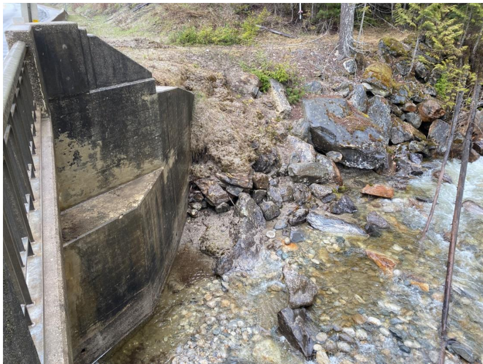
Photograph 8. View looking north (upstream) at the upstream wing wall of the west abutment (Photograph by BGC taken on April 26, 2023).
