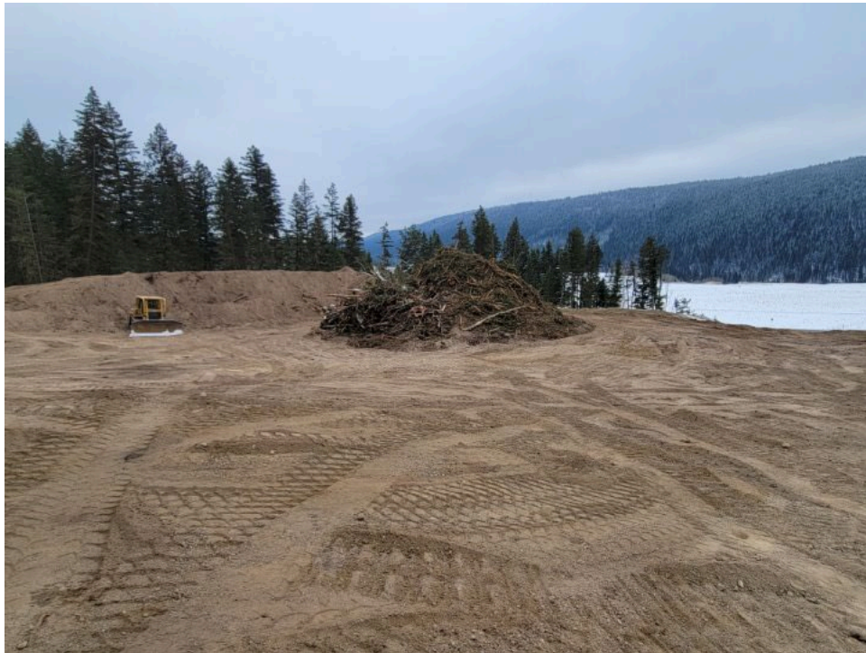
View of potential crusher set up area, looking southwest, December 2022.
